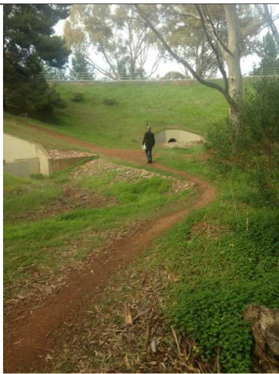
Plate 25 Bank across watercourse with culverts, minor scour
