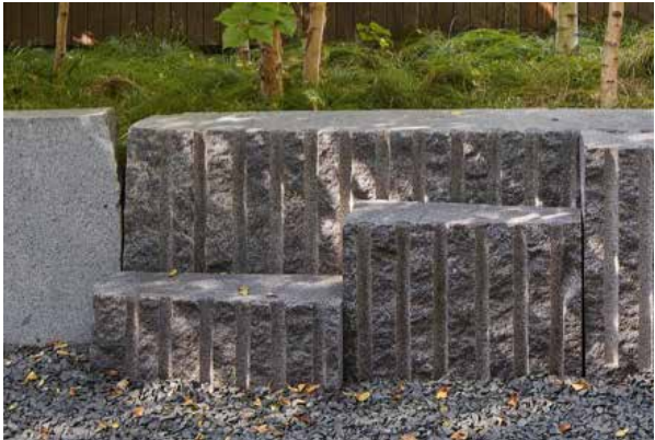
Granite Block Wall with Rusticated Edge Colour: Adelaide Black Application: Retaining and Seating wall
