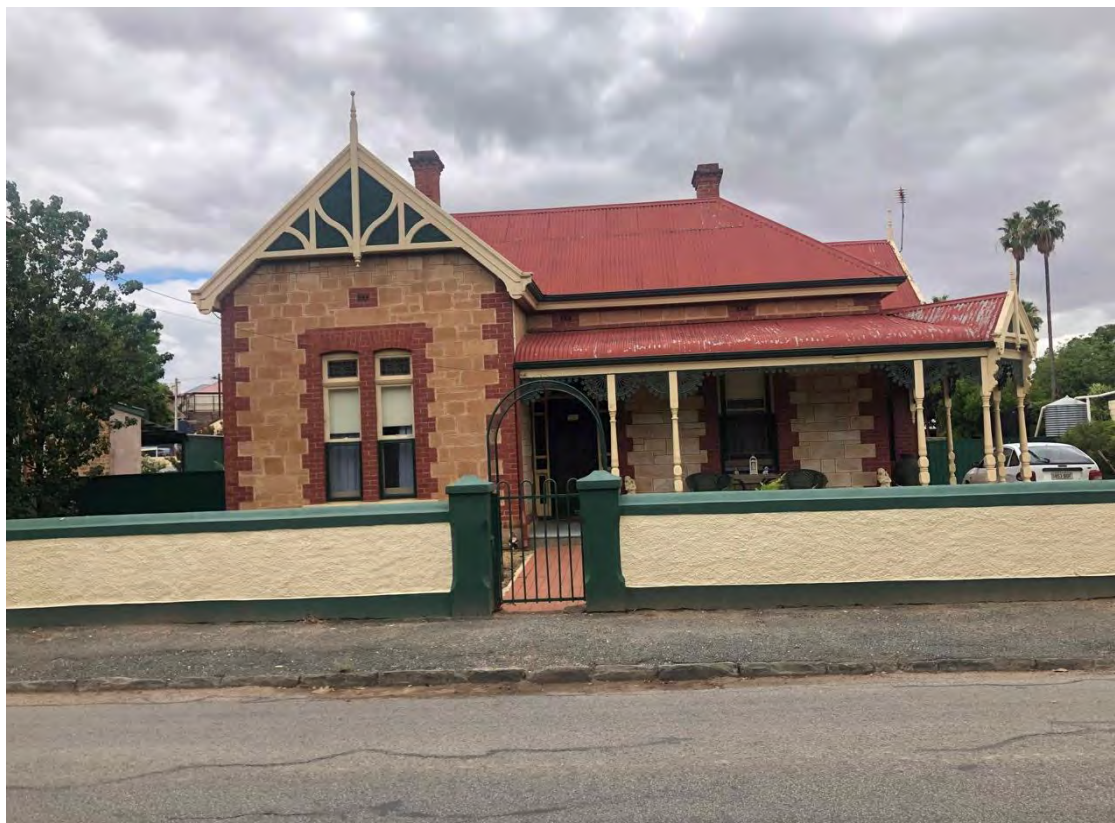
Dwelling and wall at 23 Jacob Street from south
