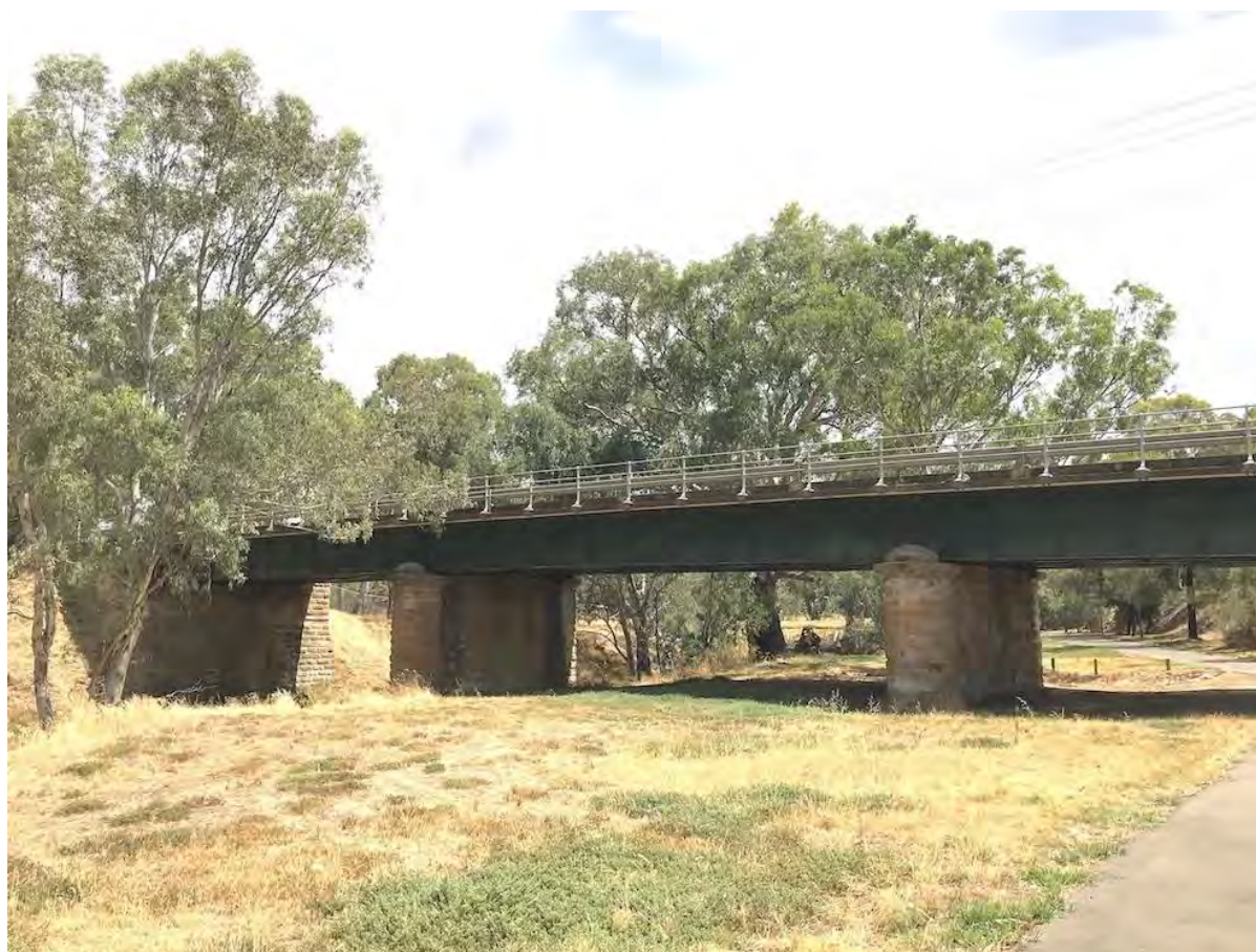
Willaston Bridge, looking north
