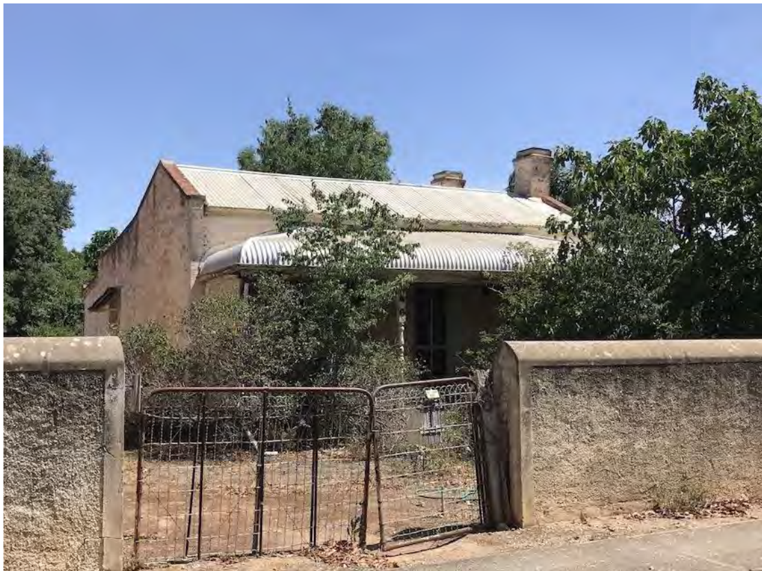
Dwelling and Wall at 6 Twenty-First Street from north
