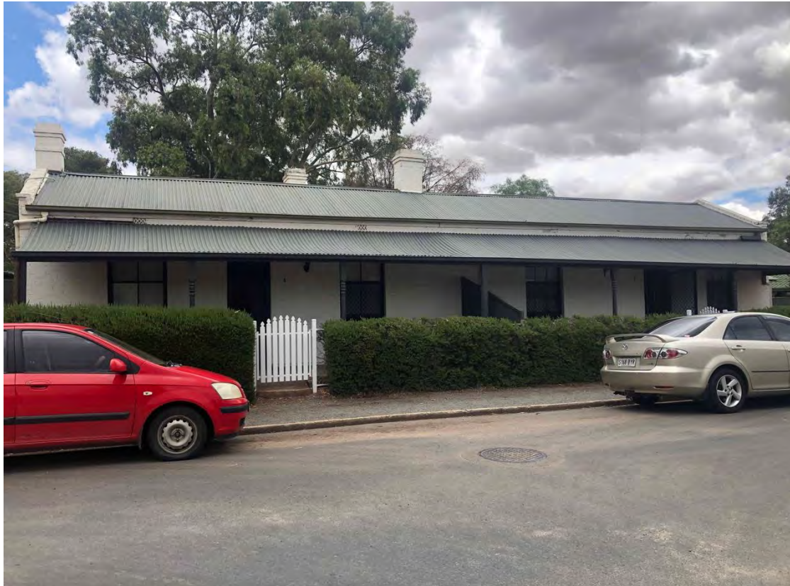
Attached dwellings at 4-6 Cameron Street from east
