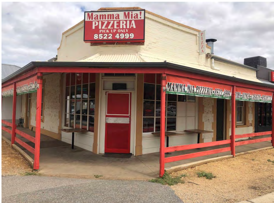
Shop at 36 Adelaide Road from north
