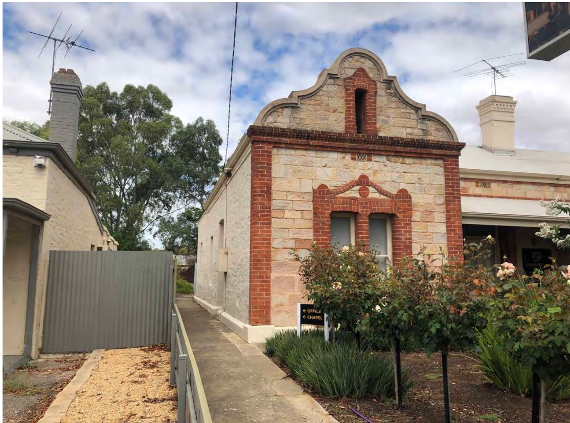
Former attached dwelling at 22a Adelaide Road from north
