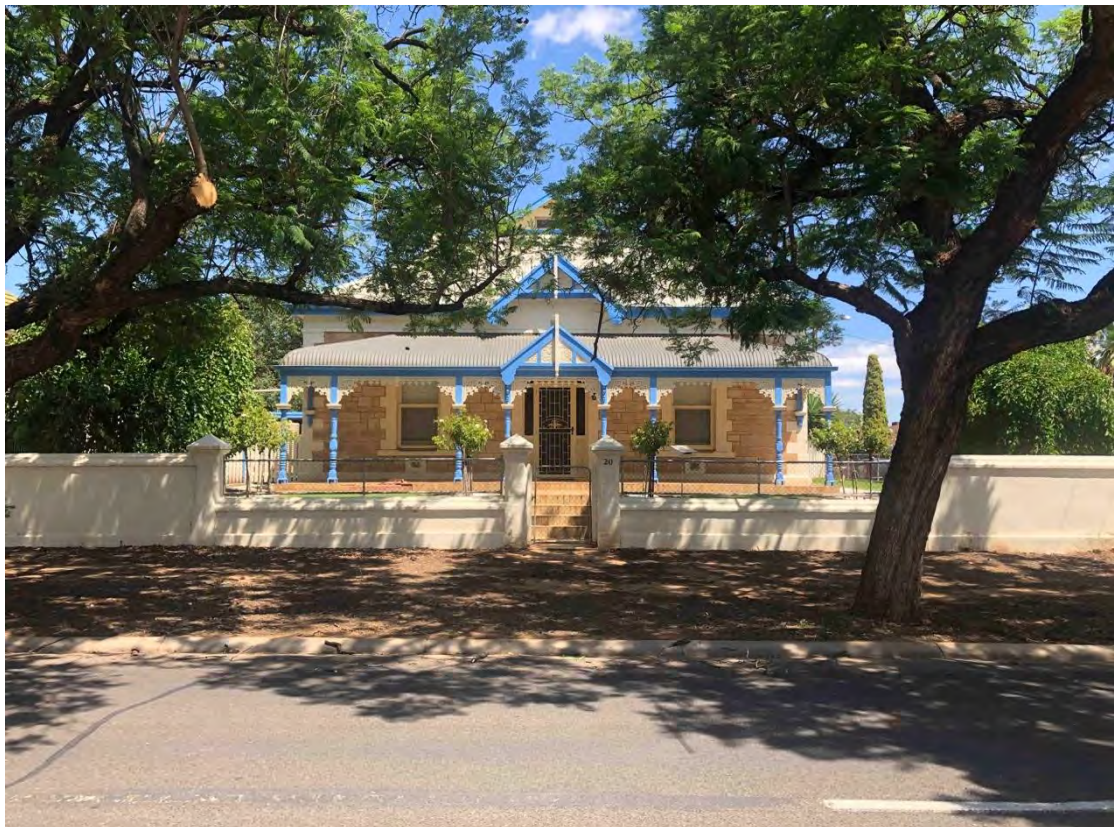
Dwelling and wall at 20 Thirteenth Street from east
