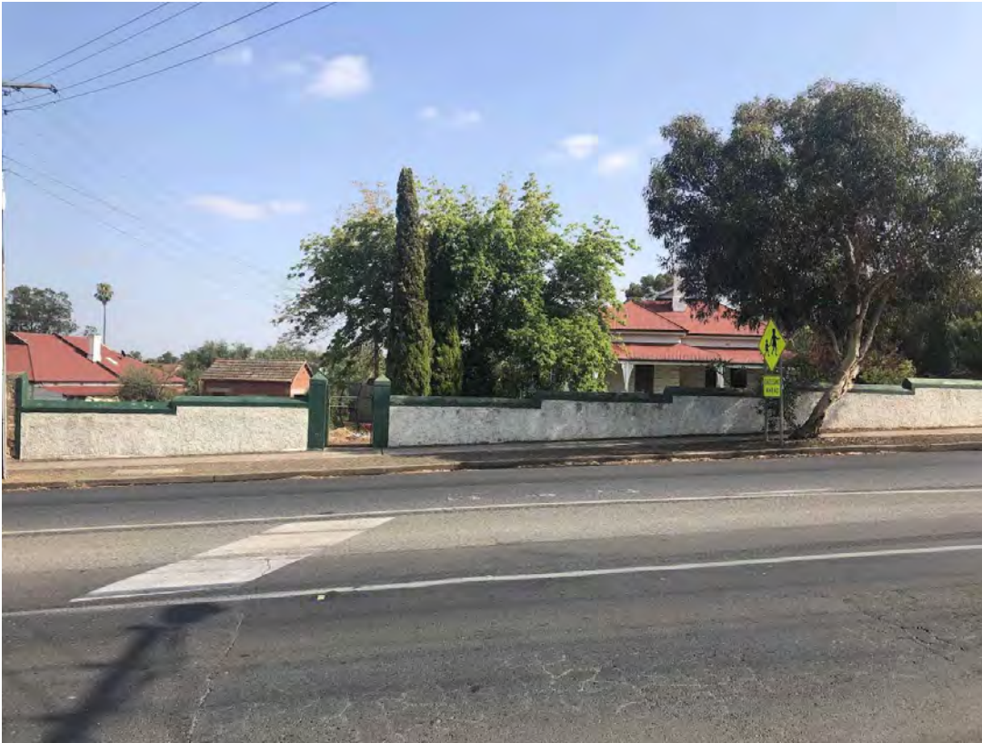
Rendered wall at 6-8 Lyndoch Road from south
