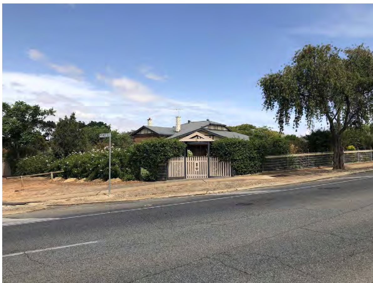
Dwelling at 32 Redbanks Road from east
