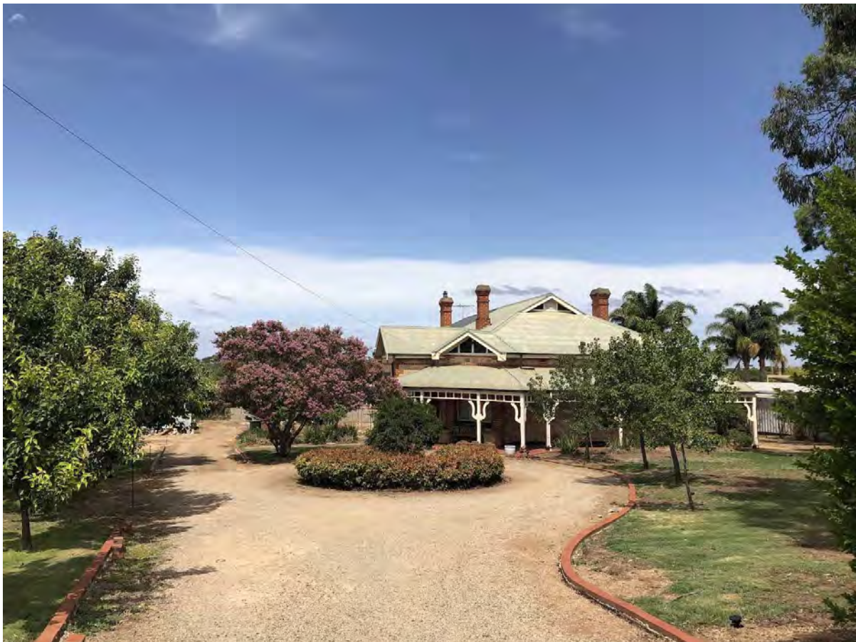
Dwelling at 40 Redbanks Road from north-east
