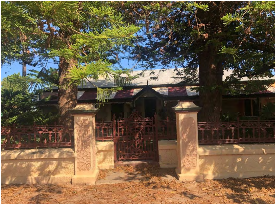
Dwelling and wall at 1 Second Street from south-east
