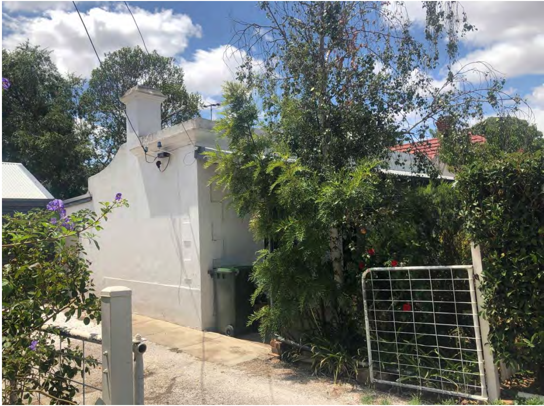
Dwelling at 8 Ninth Street from west
