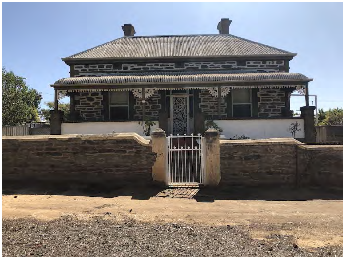
Dwelling and Wall at 22 Thirteenth Street from east
