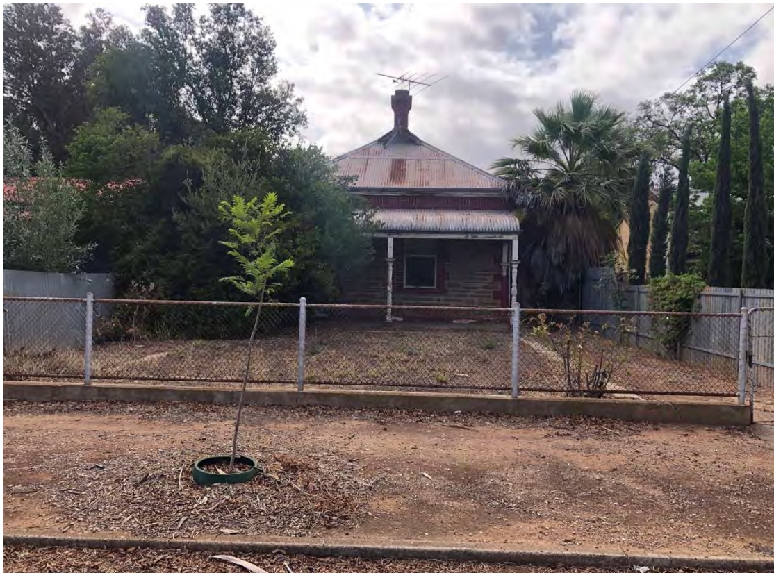
Dwelling at 21 Second Street from south-east
