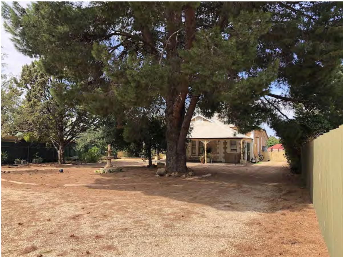
Dwelling at 46 Redbanks Road from north-east
