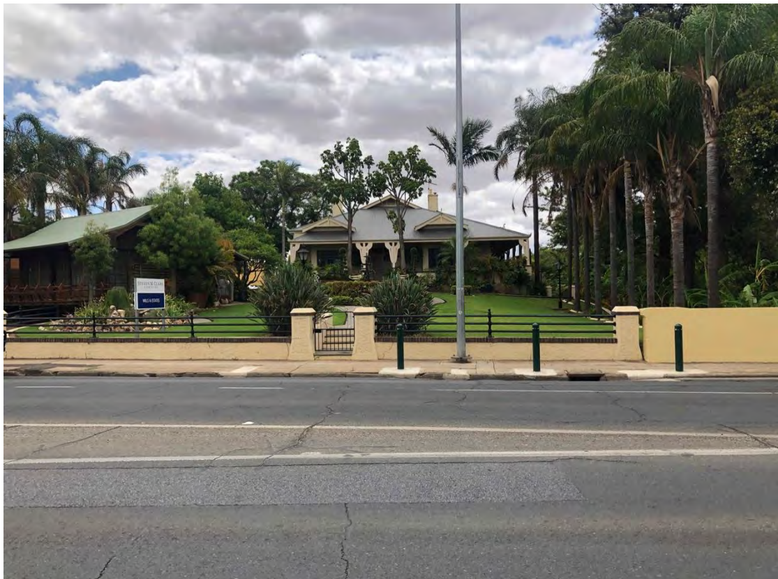
Former dwelling at 1 Adelaide Road from south-east
