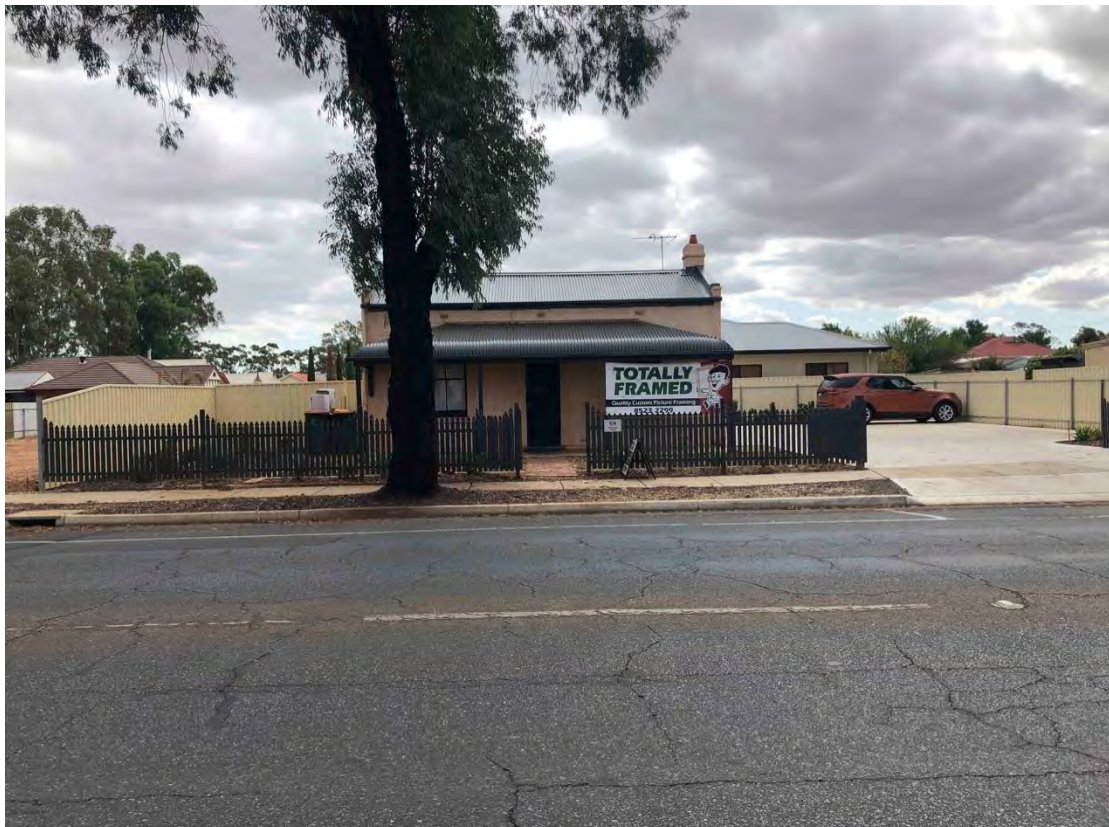
Dwelling at 59 Adelaide Road from east
