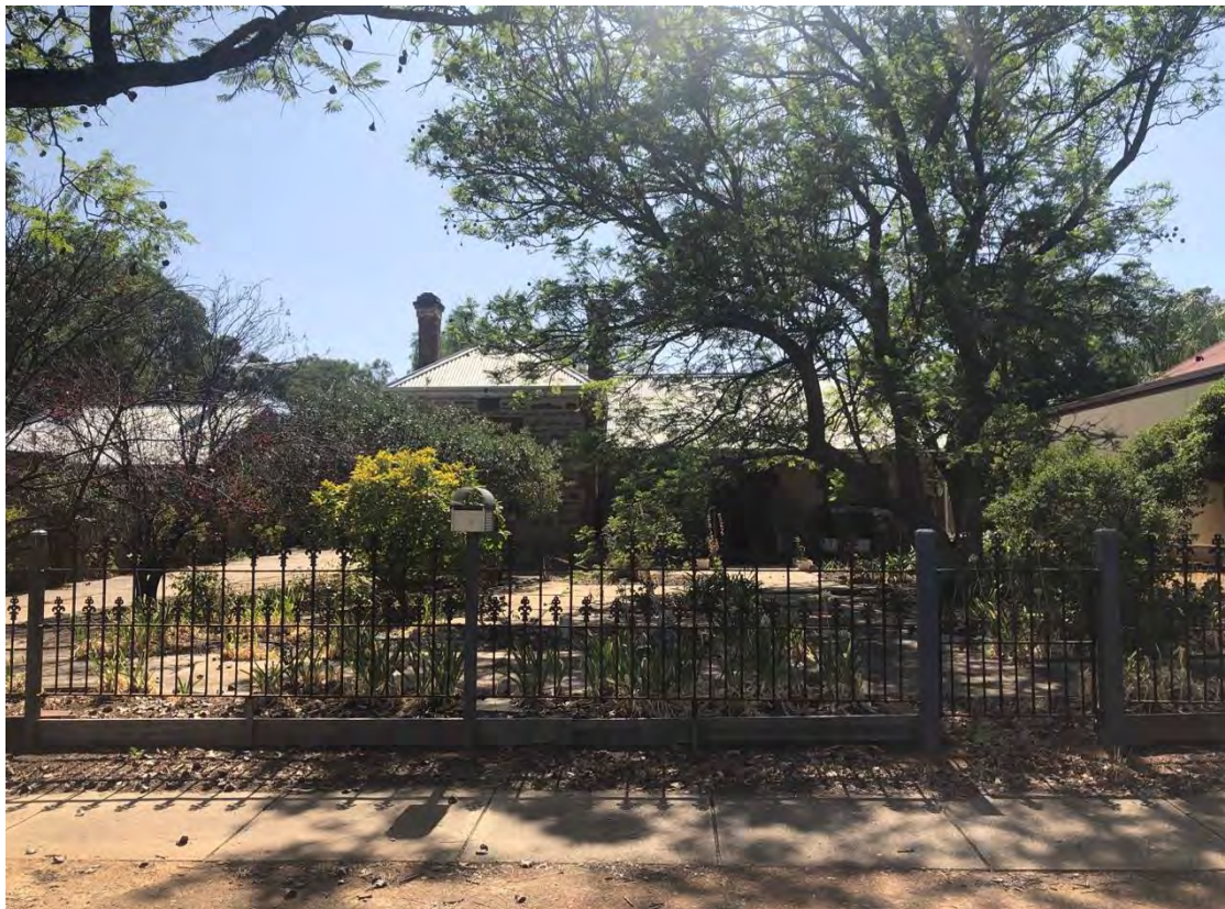
Dwelling at 20 Seventh Street from west
