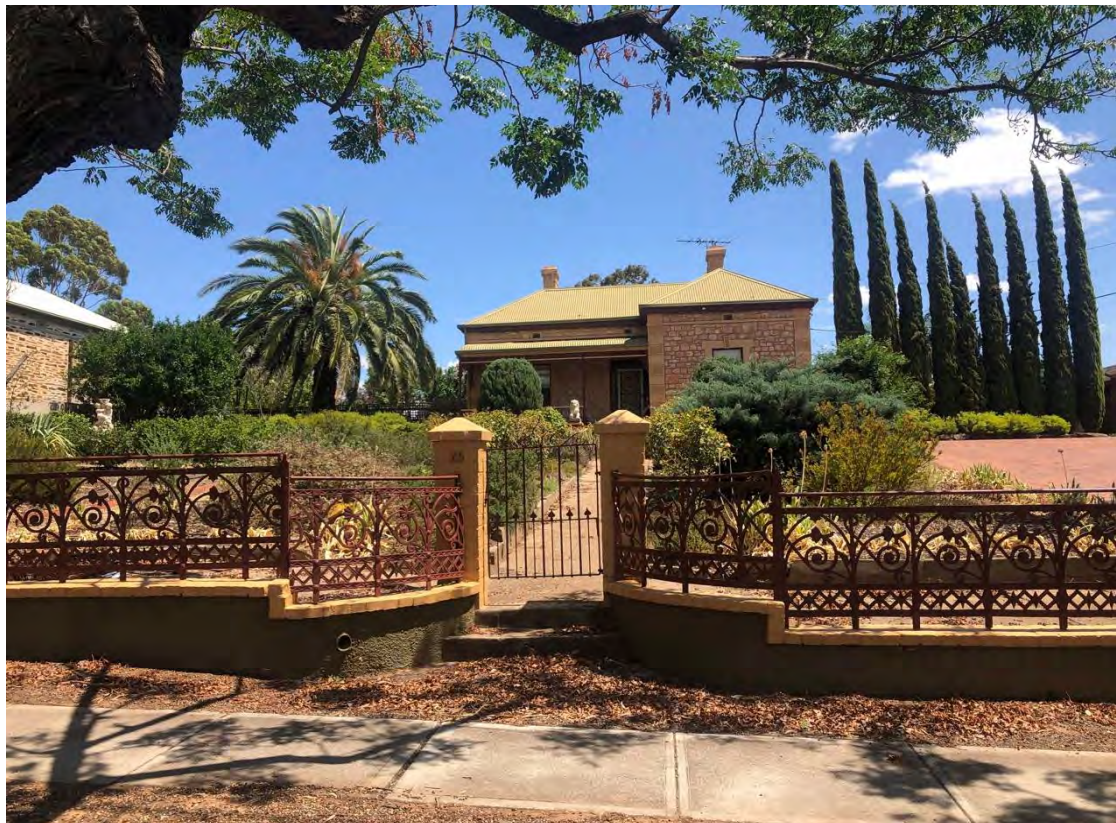
Dwelling at 26 Eighth Street from south-east
