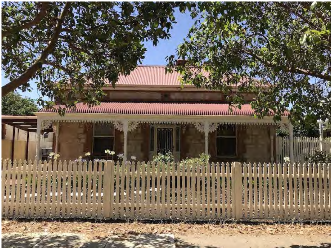
Dwelling at 5 Twenty-First Street from south
