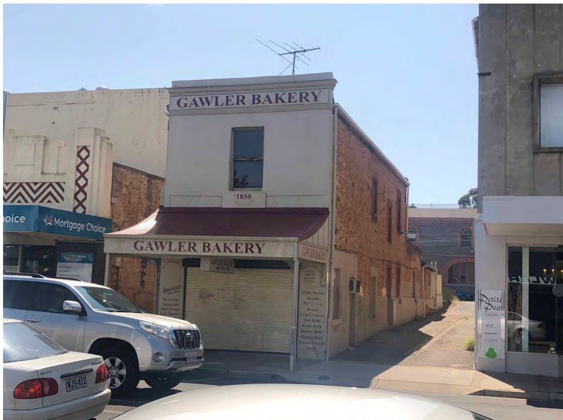
Shop and residence at 65 Murray street from west
