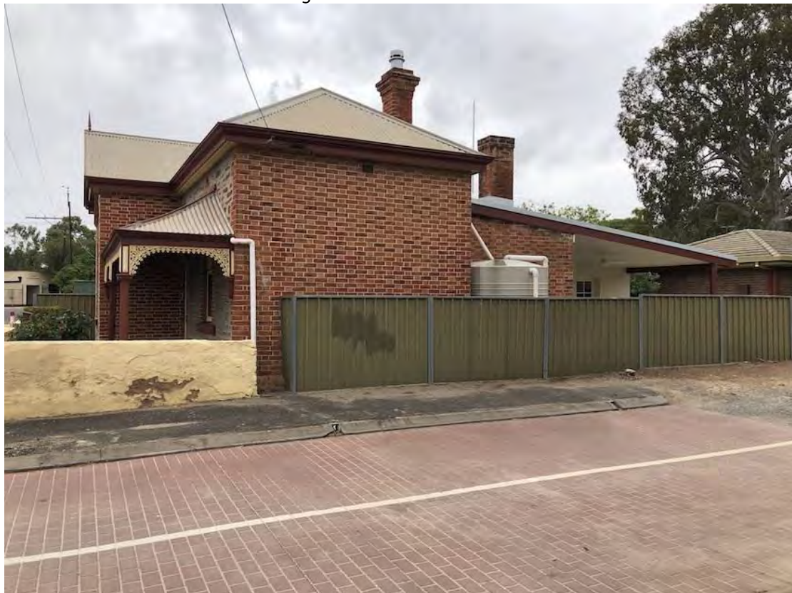
Dwelling at 13 Howard Street from south, indicating distinctive brick walling
