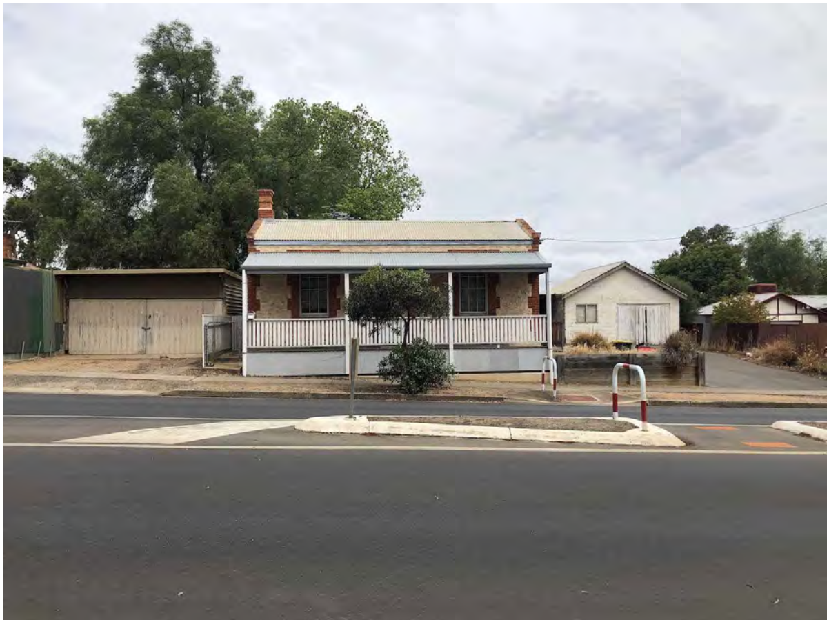
Dwelling at 49 Paxton Street from north-west
