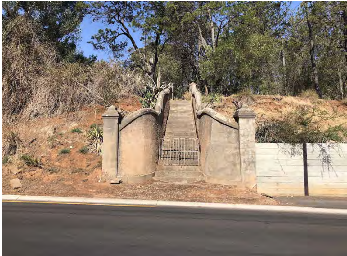
Entrance stairs at 6 Duffield Street from west
