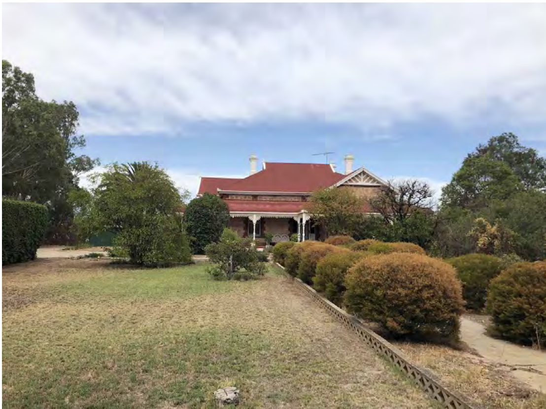
Dwelling at 50 Redbanks Road from north-east
