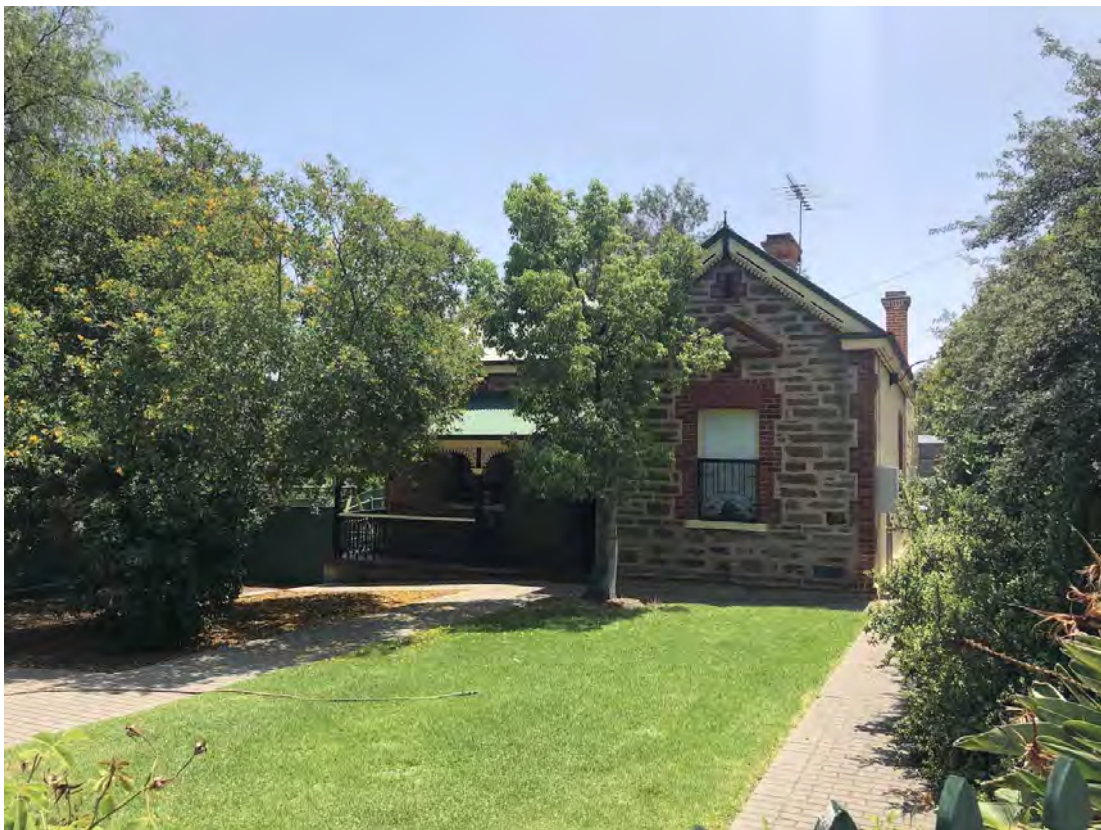
Dwelling at 2 Short Street from south-east
