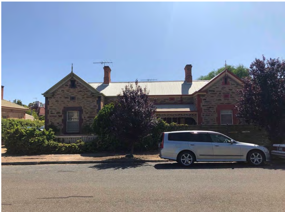
Attached dwellings at 4a-b Thirteenth Street from east
