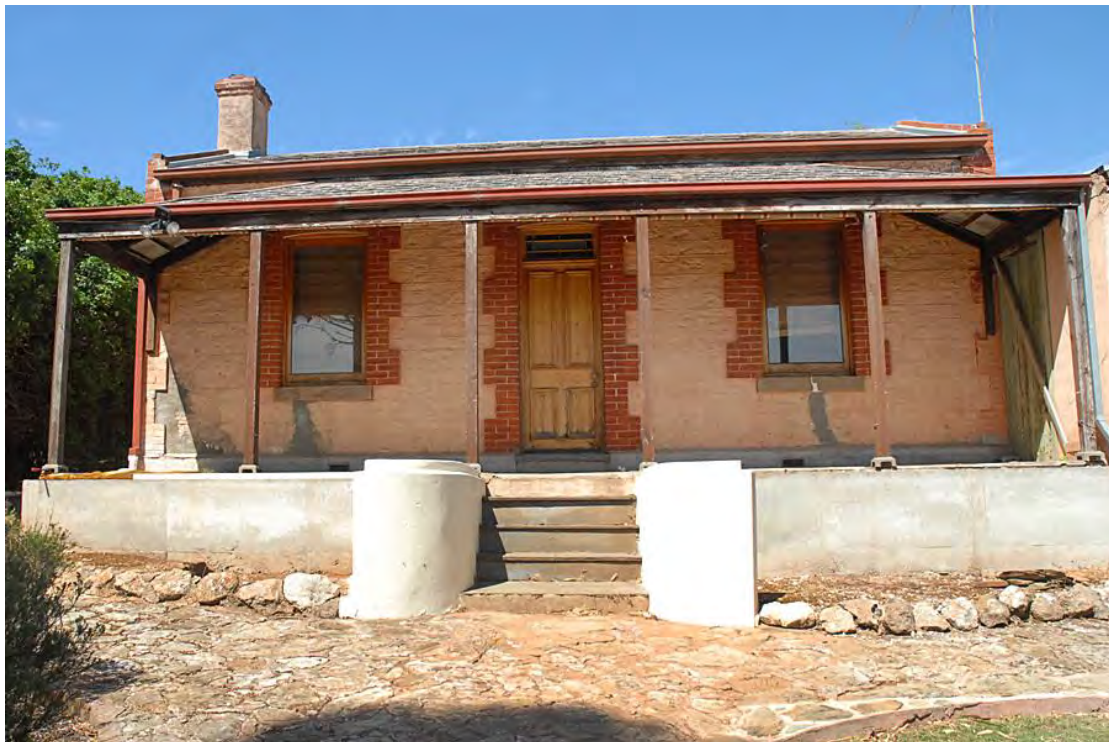
7 Duffield Street, Gawler East, viewed from west [Source: gawlerhistory.com]
