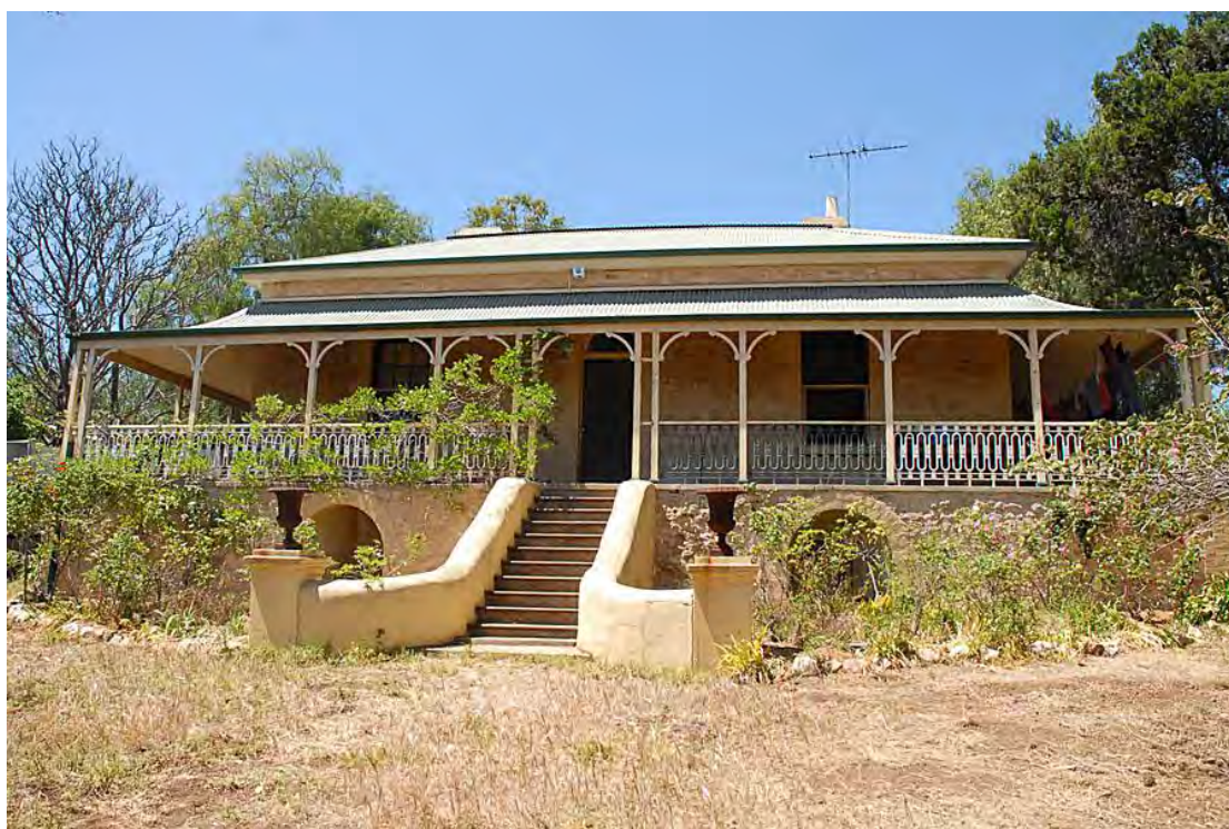
9 Duffield Street, Gawler East, viewed from west [Source: gawlerhistory.com]
