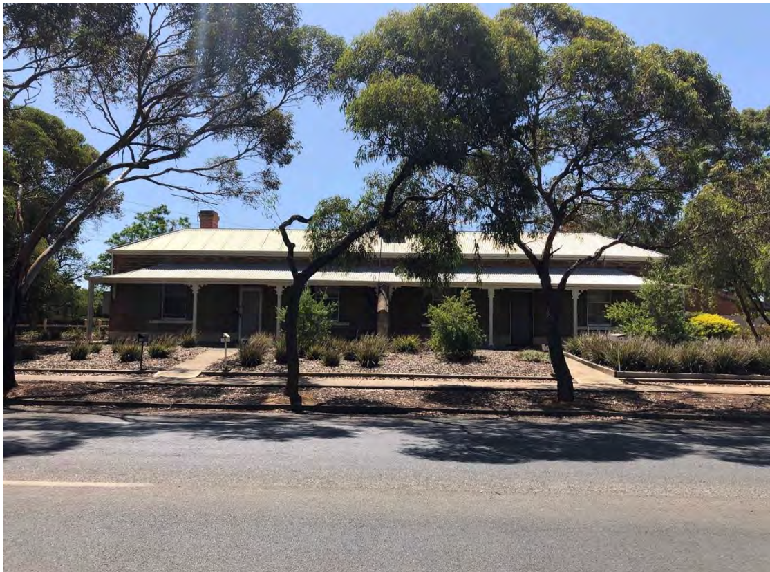
Dwelling at 17-17a and 19-19a Twelfth Street from south-east
