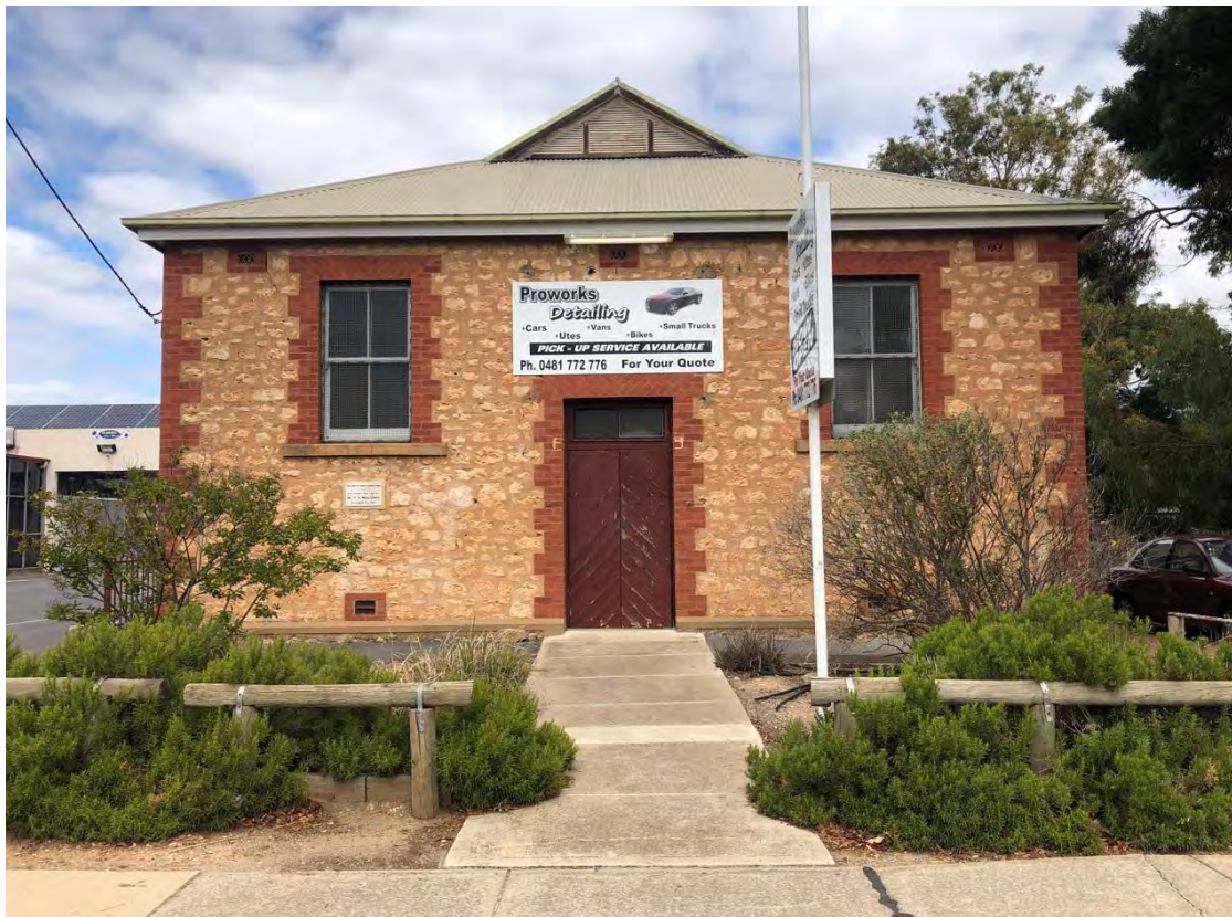
Former Church Hall at 50 Adelaide Road from north-west
