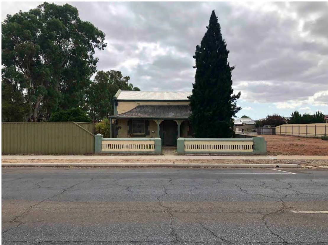
Dwelling and wall at 63 Adelaide Road from east
