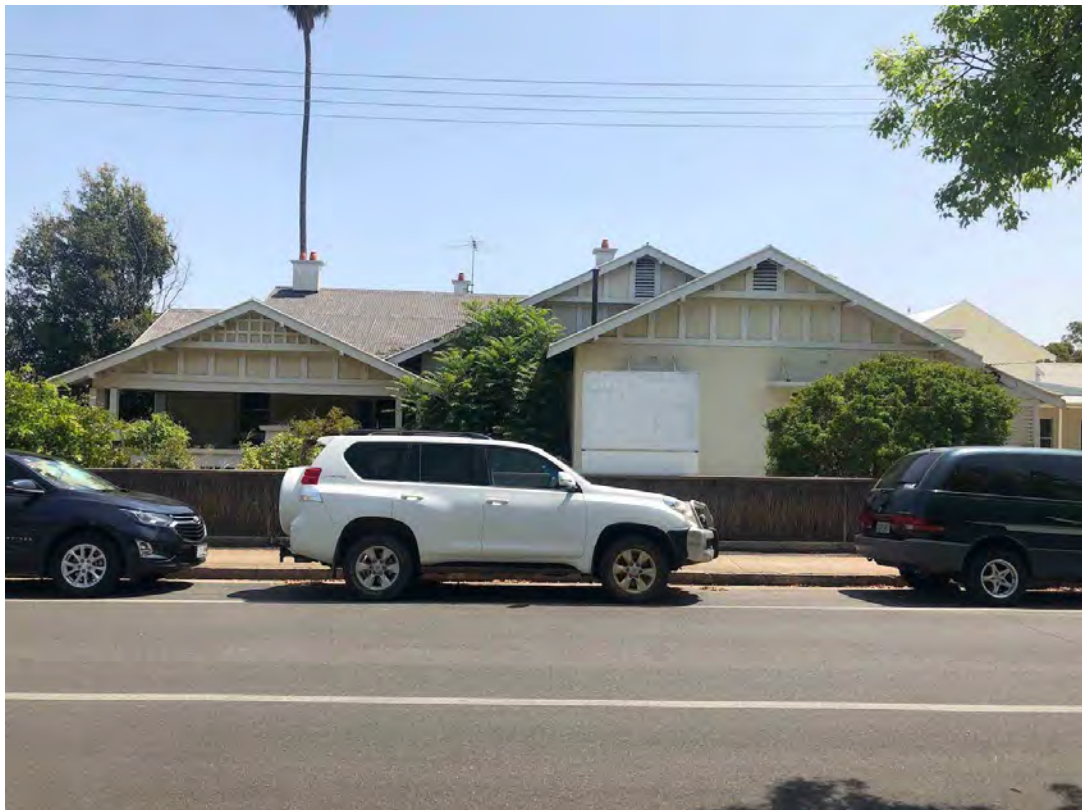
Dwelling at 14 Union Street (1 Warren Street) from South
