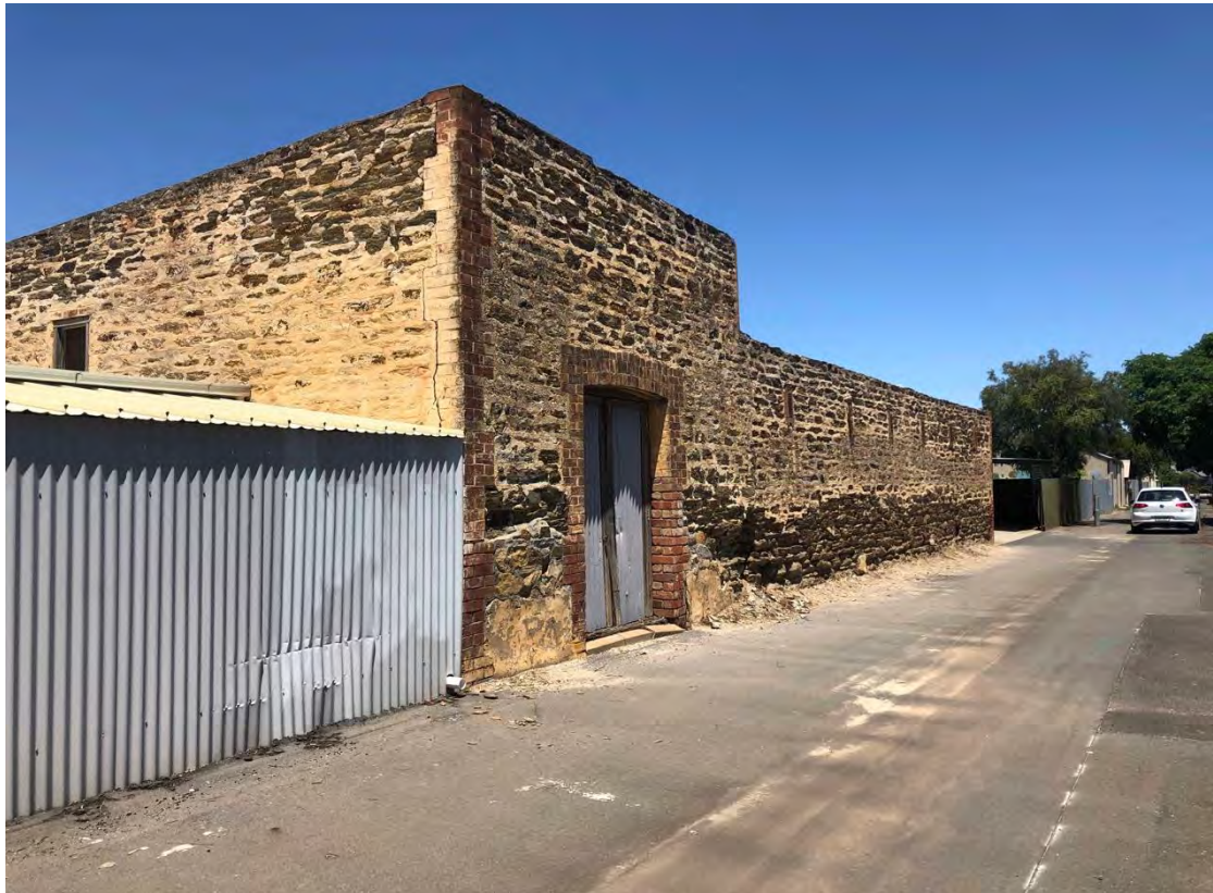
Stone Shed and Wall at rear of 27 Fourth Street from north-east
