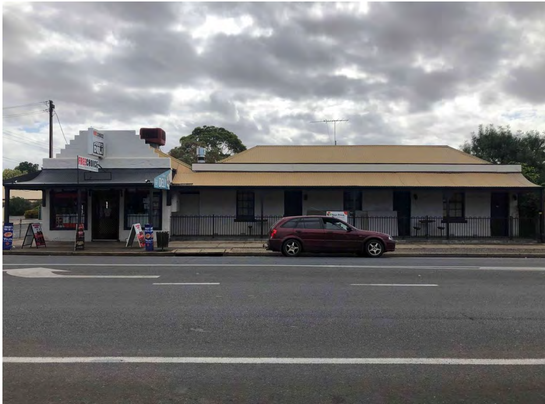
Corner shop and attached cottages at 41 Adelaide Road from east
