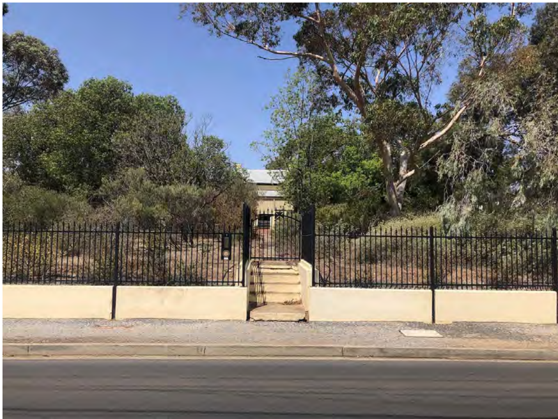
Dwelling at 1 Daly Street from west
