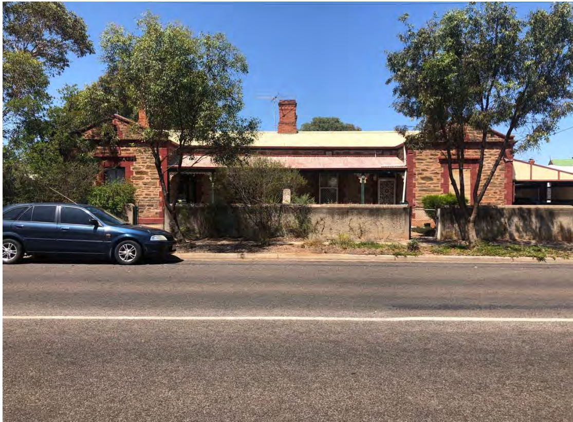
Attached dwellings and wall at 7-7a Fifth Street from north-east
