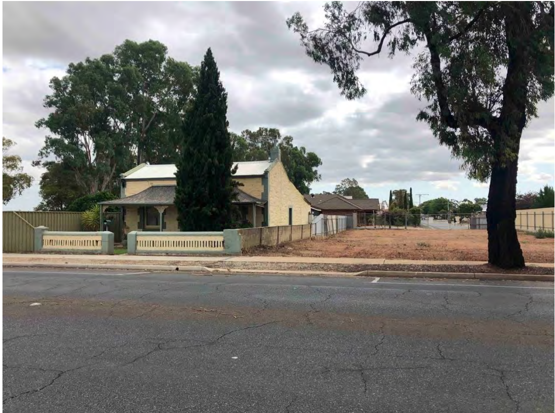
Dwelling and wall at 63 Adelaide Road from north-east
