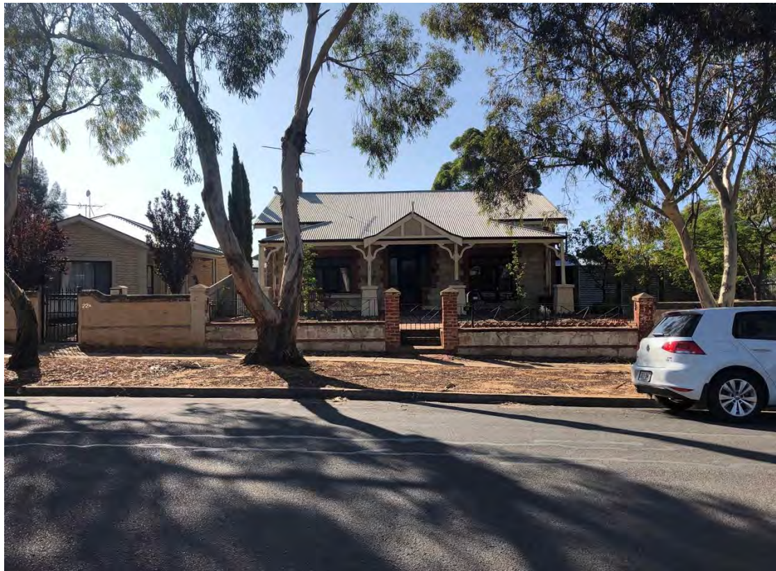
Dwelling at 22 Eighth Street from south-east
