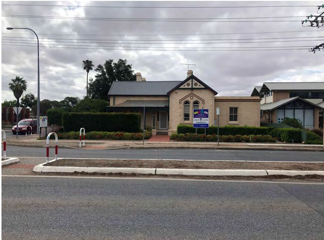
Former dwelling at 27 Adelaide Road from south-east
