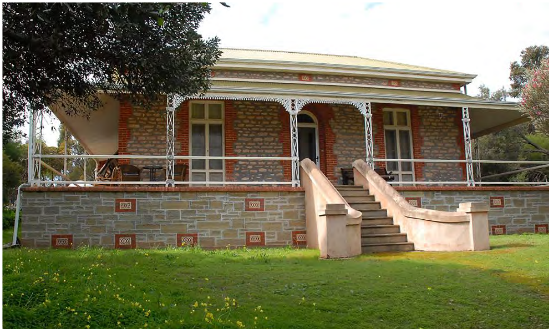
Dwelling and front wall at 7-9 Blanch from west
