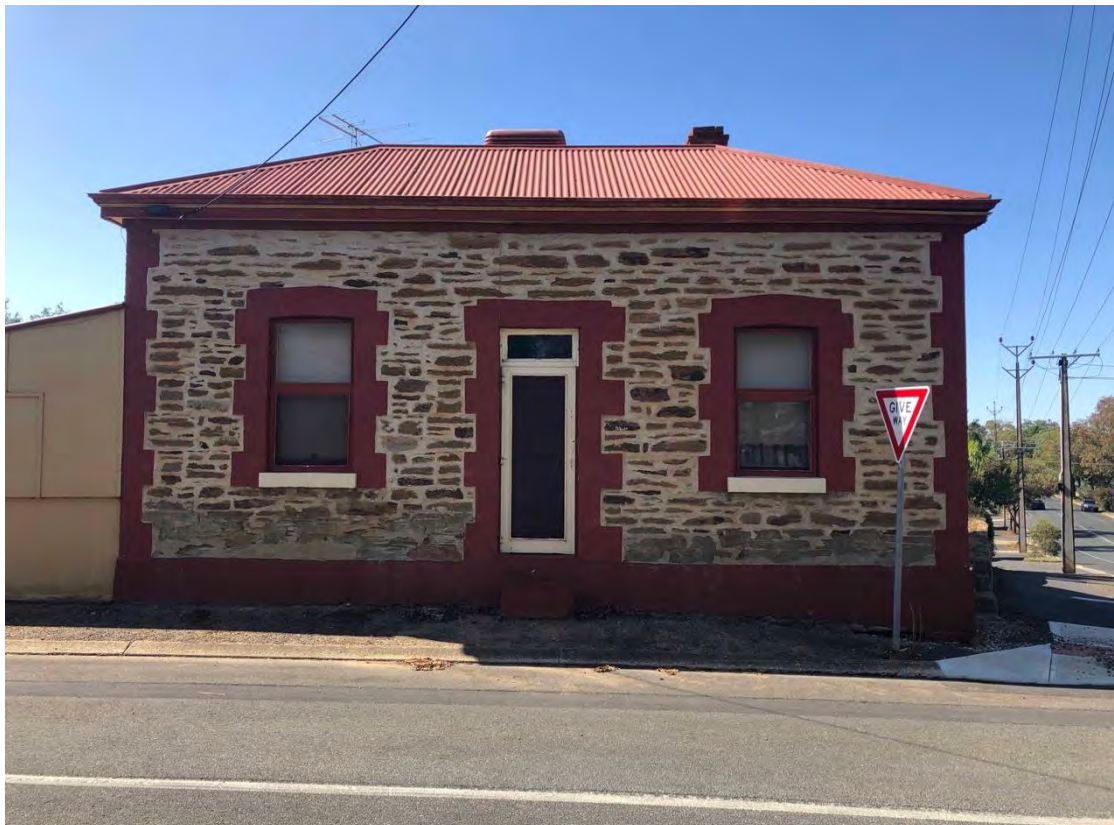
Dwelling at 3 Sixteenth Street from south
