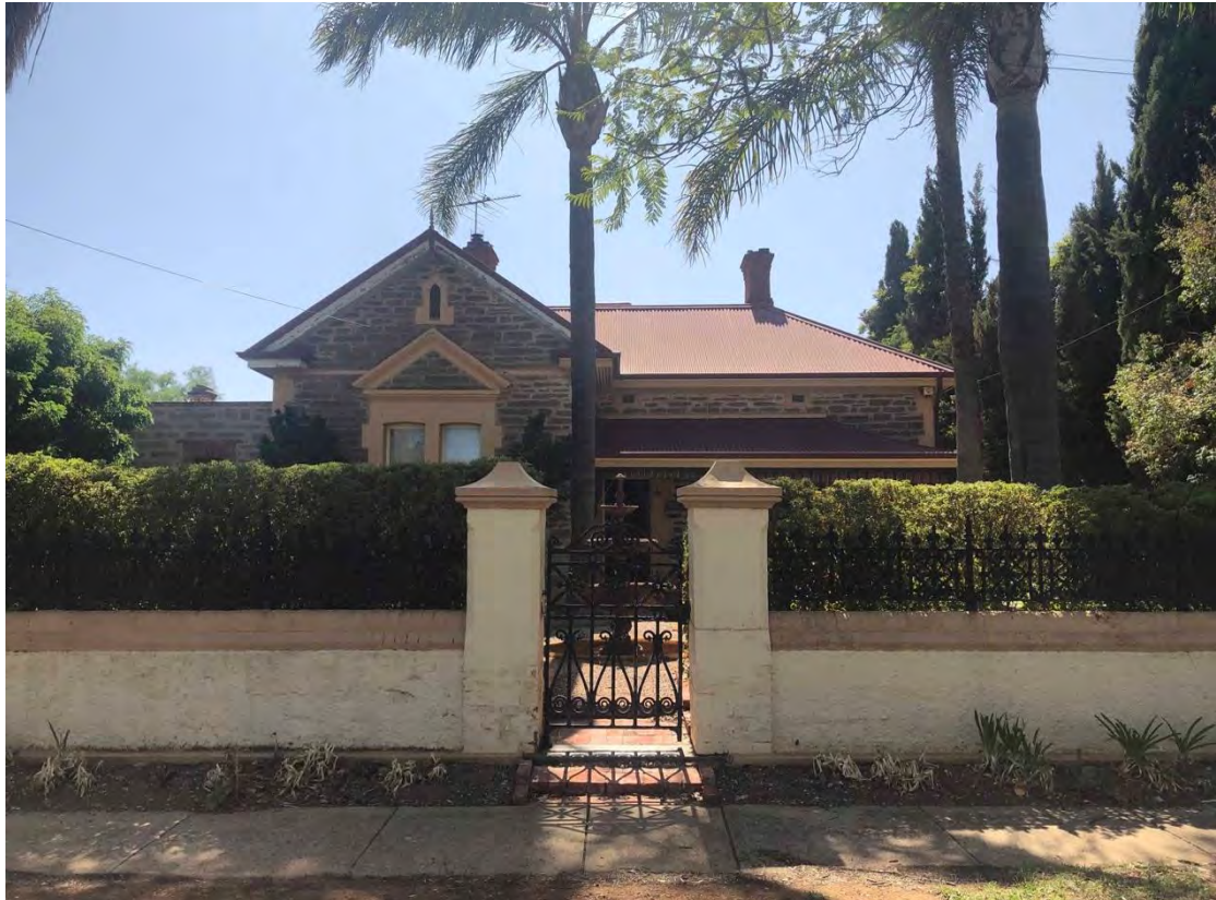
Dwelling and wall at 22 Seventh Street from west
