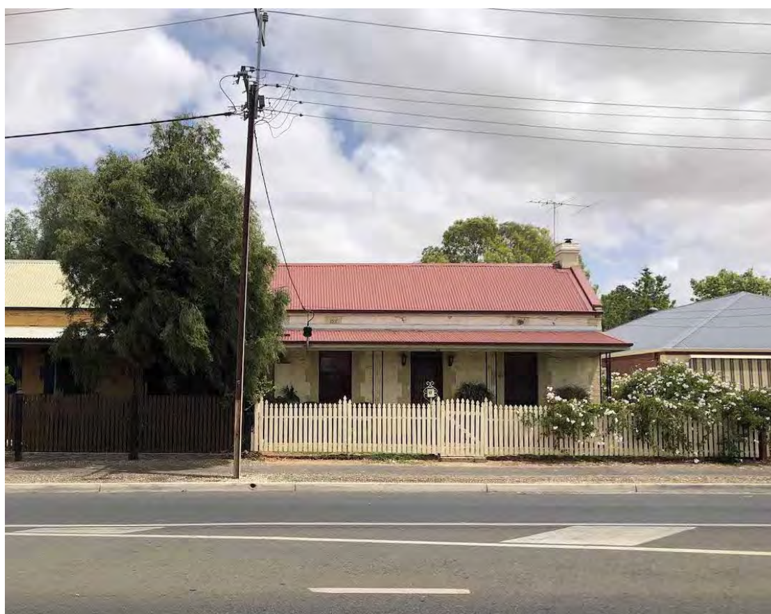
Dwelling at 40-42 Main North Road from south-east
