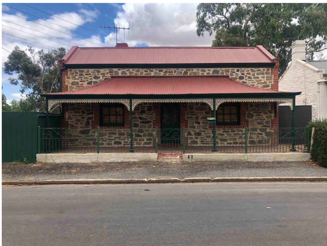
Dwelling at 2 Cameron Street from east
