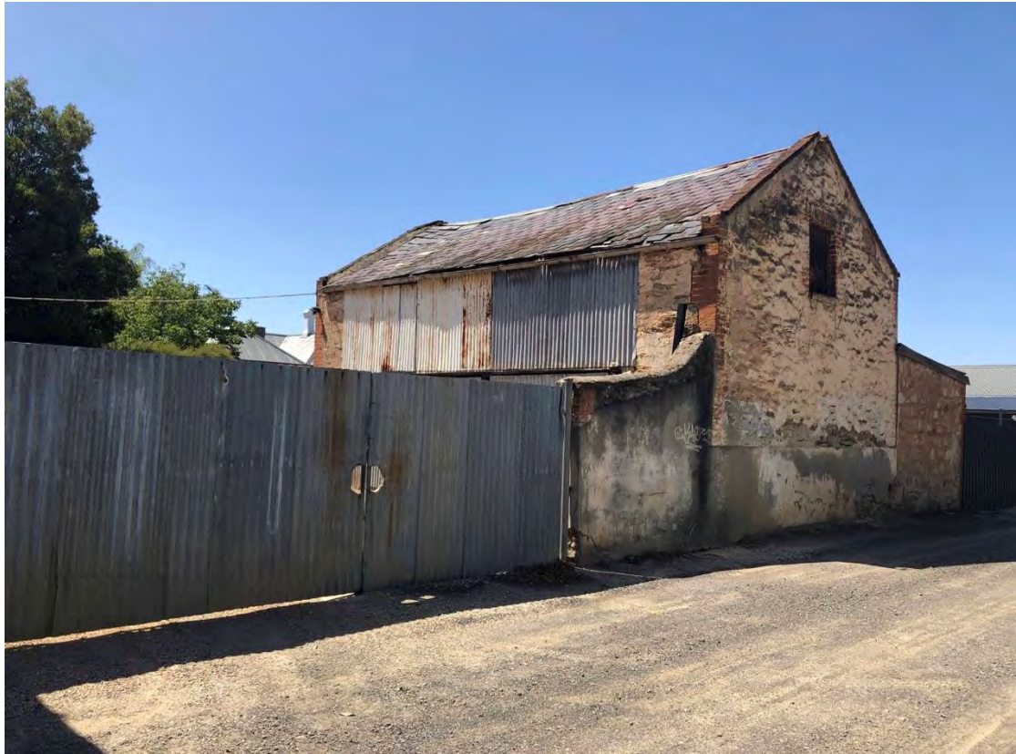
Stone outbuilding to rear of 26 Twelfth Street from south-west
