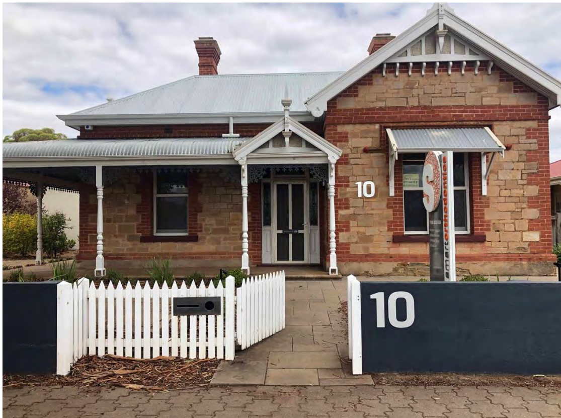
Former dwelling at 10 Adelaide Road from north-west
