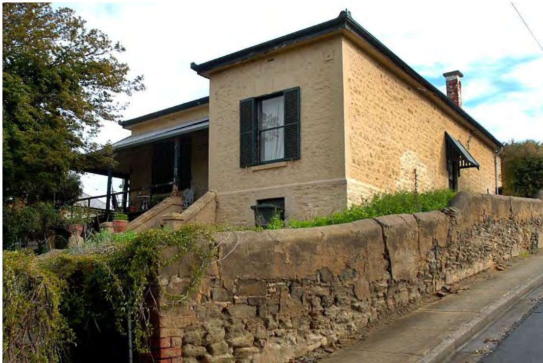
Dwelling at 6 Calton Road from south
