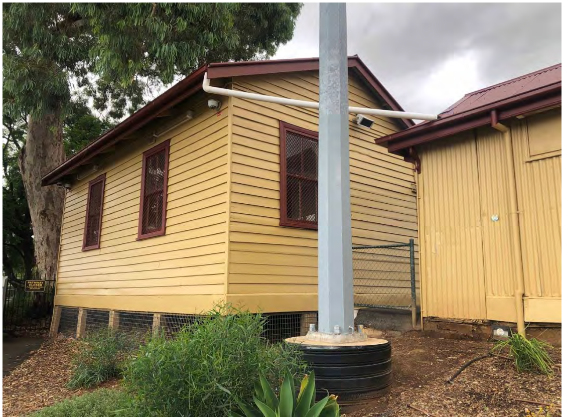
Railway Station ticket office building from north-west
