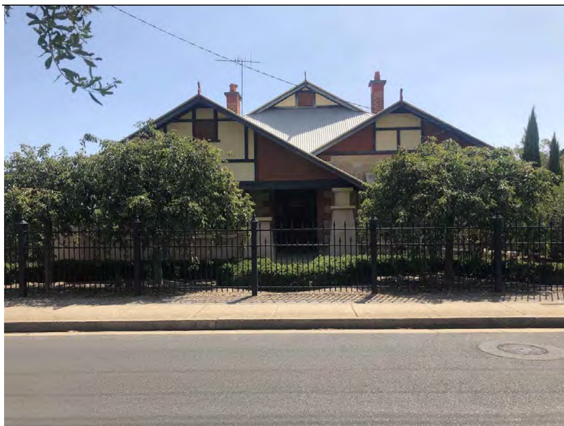
Dwelling at 6 Daly Street from east
