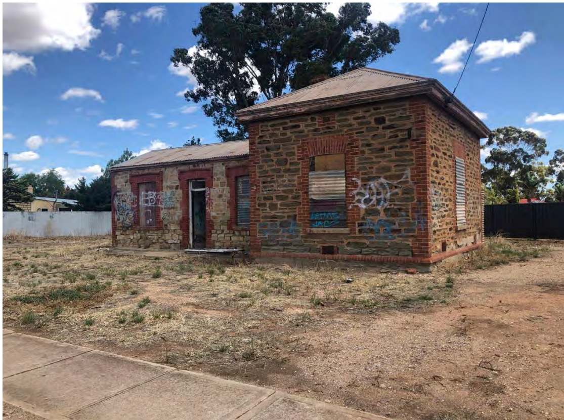
Dwelling at 17 Barnet Road from north-east
