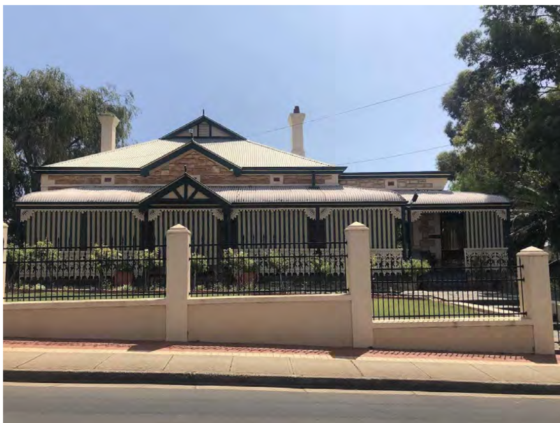
Dwelling at 22 Daly Street from east
