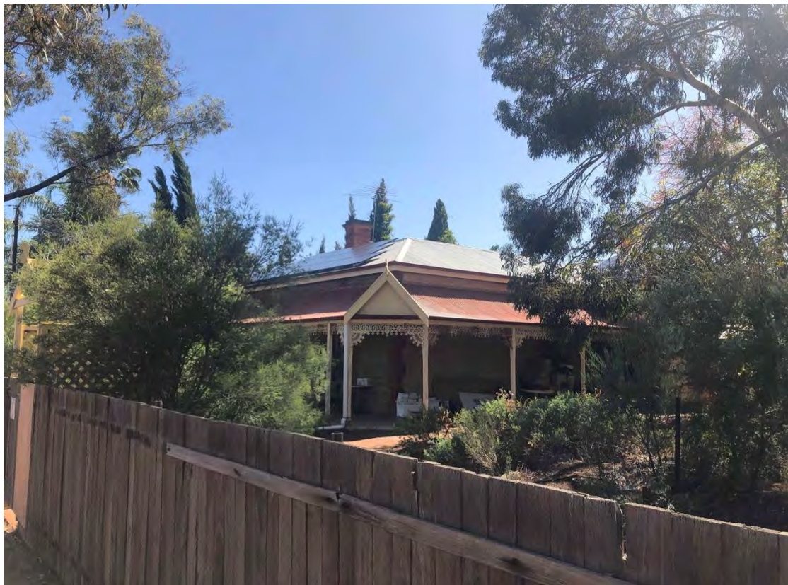
Dwelling at 24 Seventh Street from west
