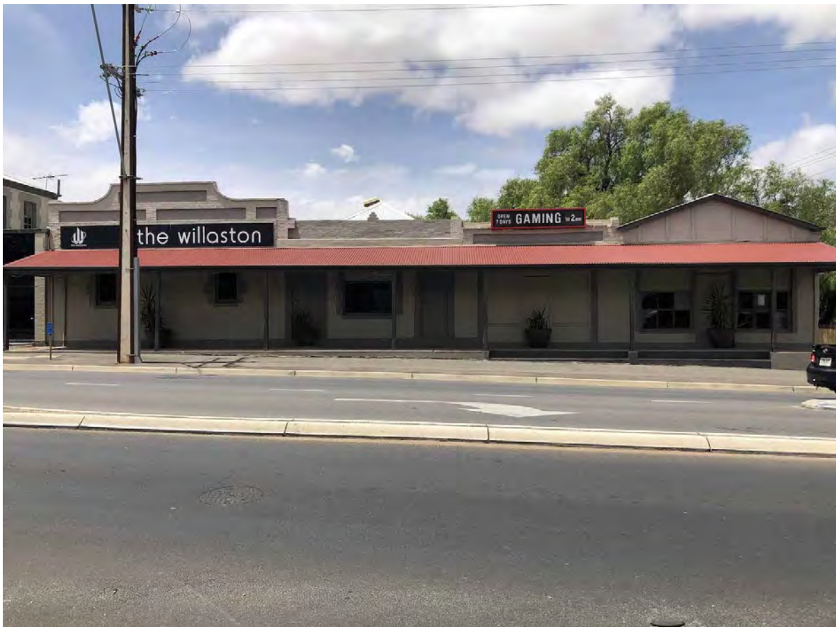
Shops at 25-29 Main Street from west
