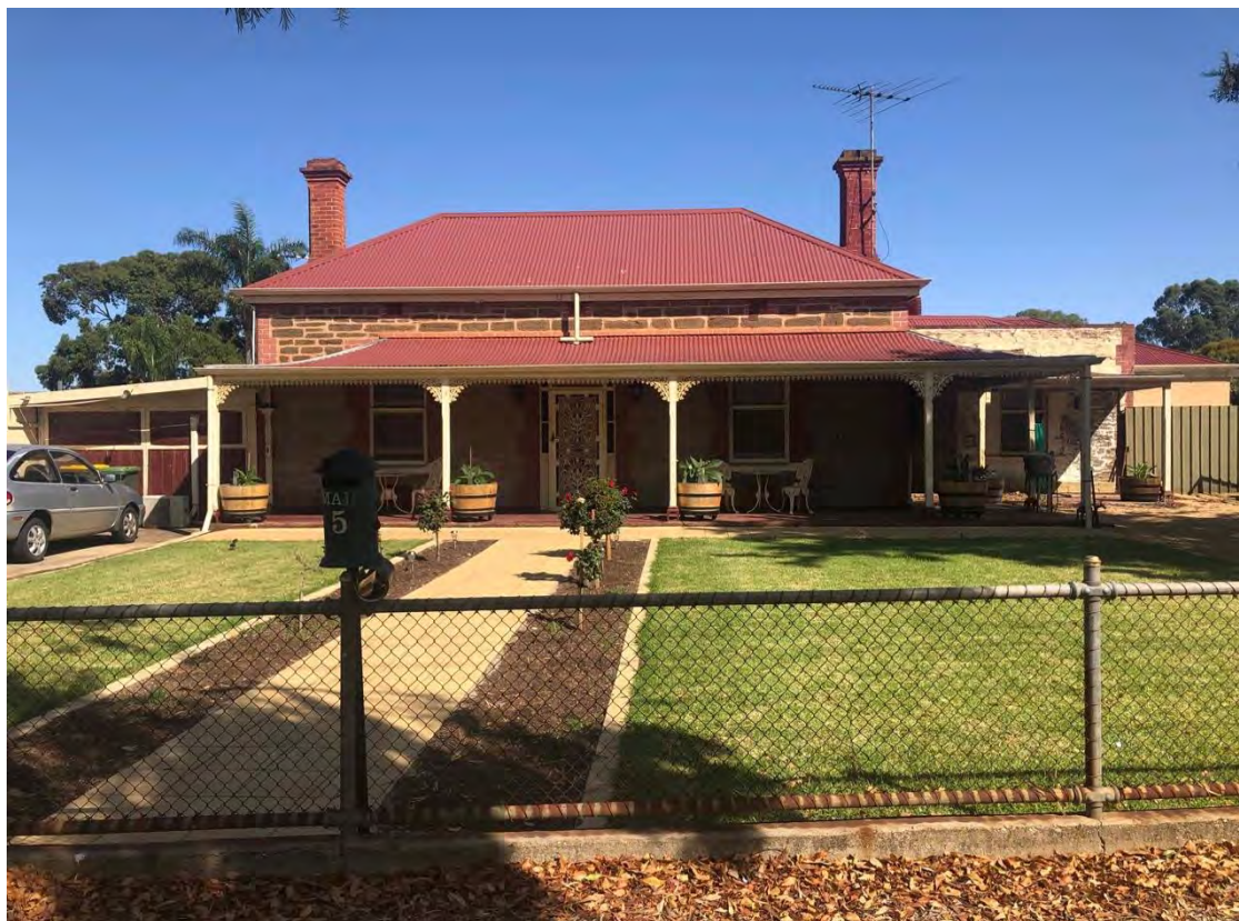
Dwelling at 5 Second Street from south-east
