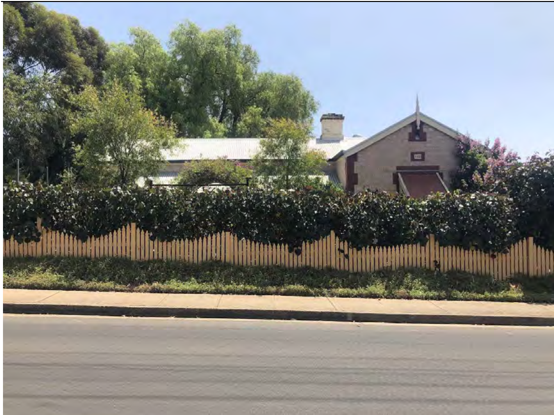
Dwelling at 26 Daly Street from east
