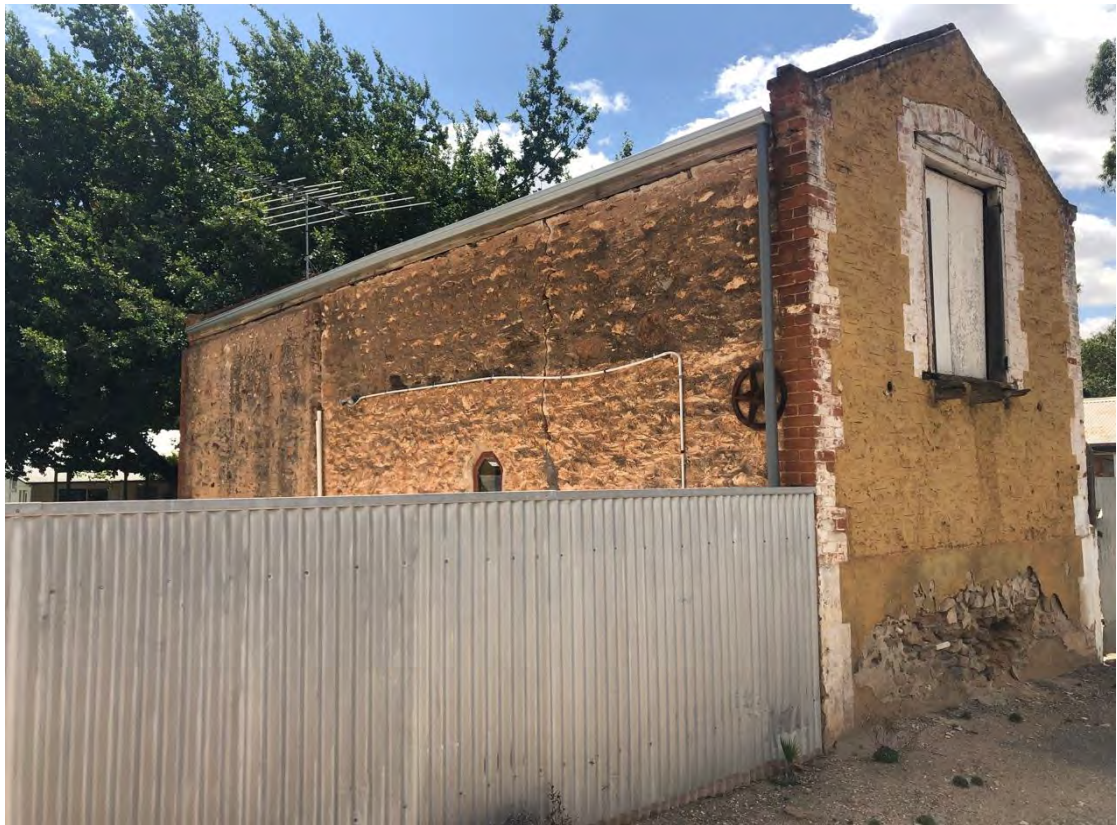
Former stable to rear of 30 Fourth Street (Cross Lane)
