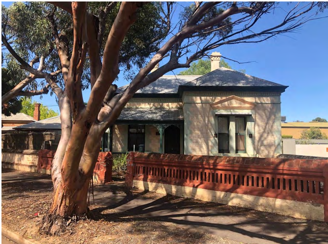
Dwelling and wall at 1 Seventh Street from north-east
