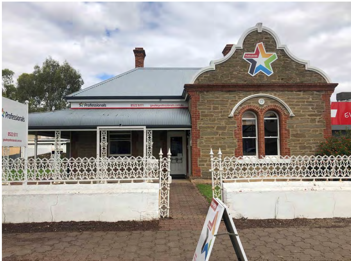
Former dwelling at 32 Adelaide Road from north-west
