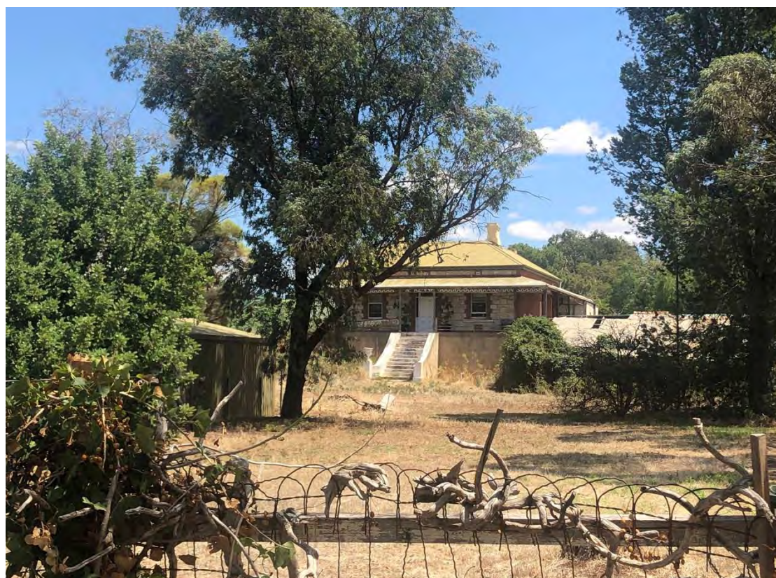
Dwelling at 34 Eighth Street from south-east
