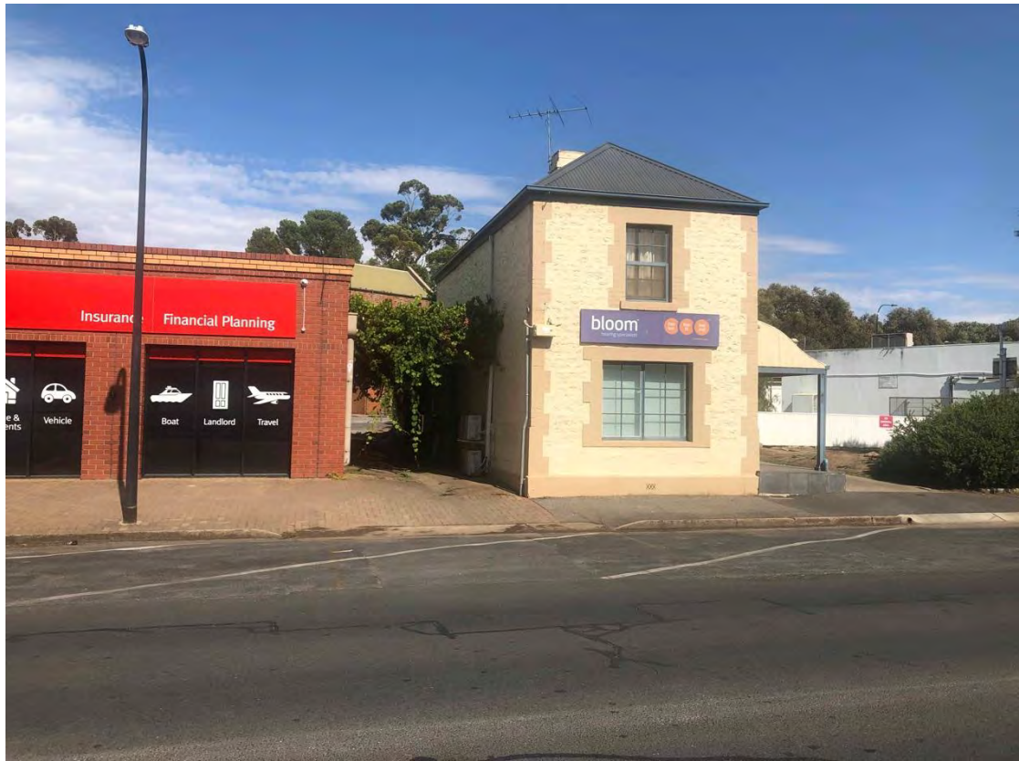
Former dwellings at 8 Murray Street from east
