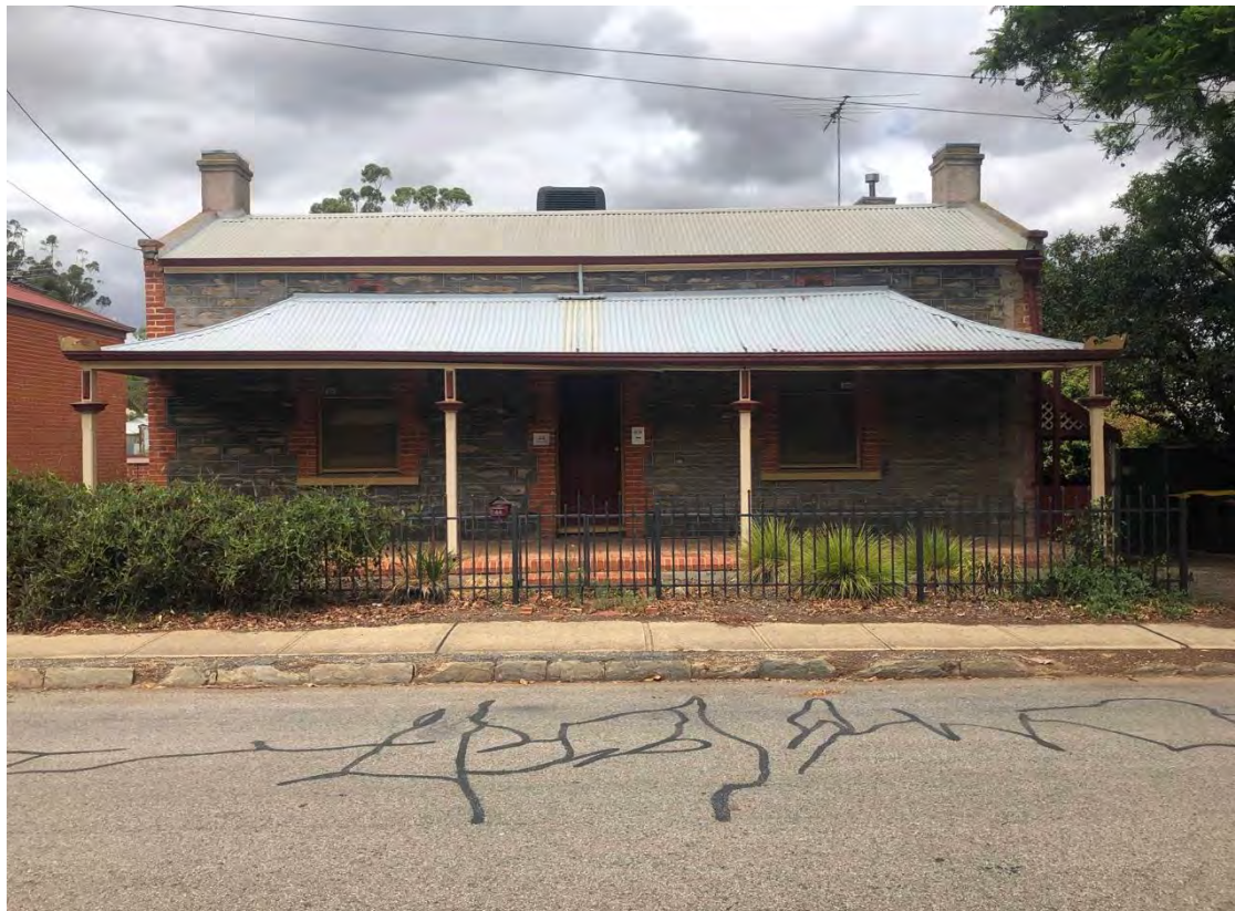
Dwelling at 44 Jacob Street from north
