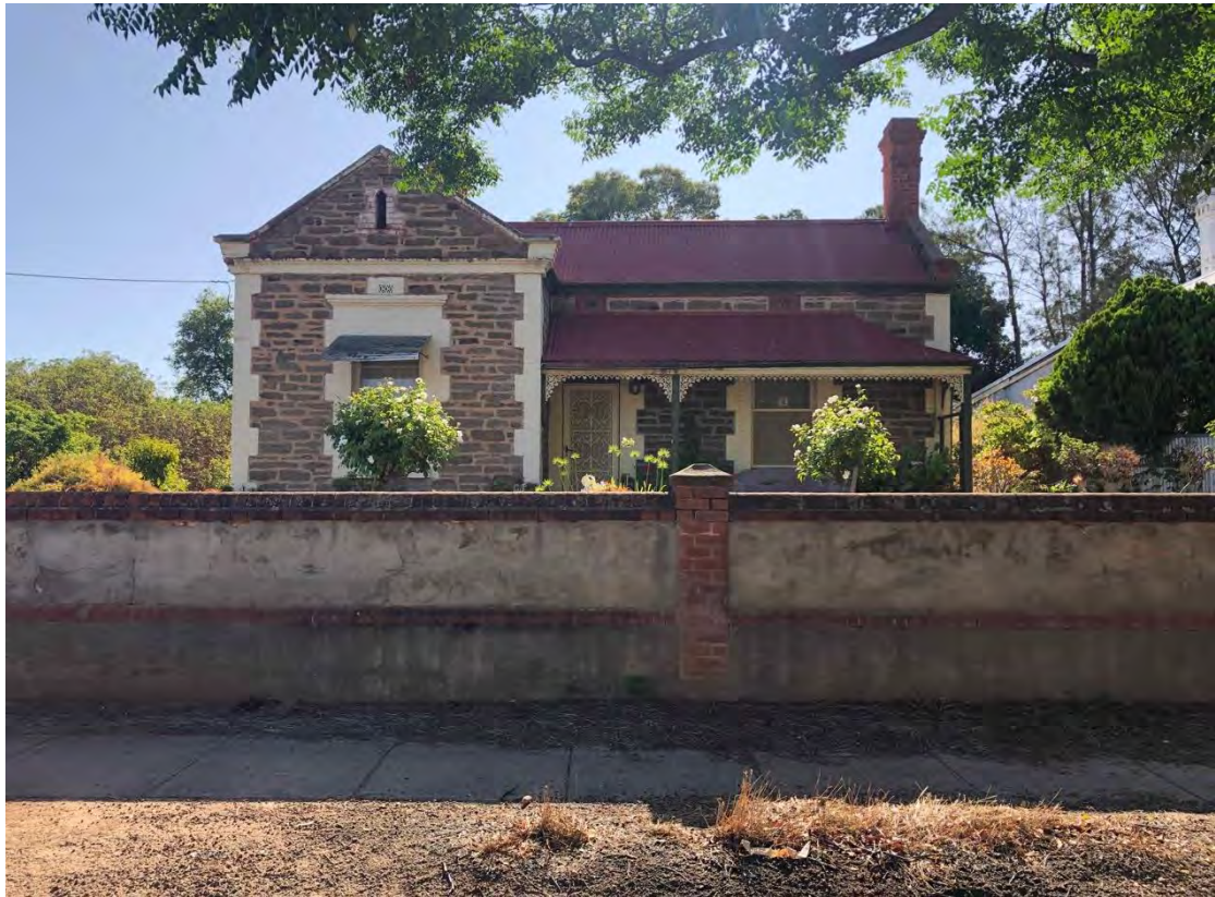
Dwelling and wall at 16 Eighth Street from east
