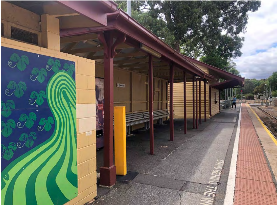
Railway Station shelter building from west
