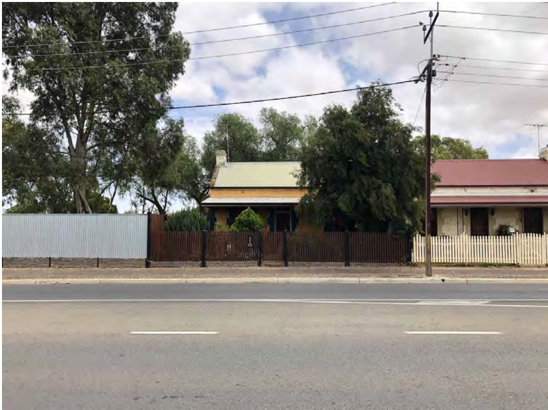
Dwelling at 40-42 Main North Road from south-east
