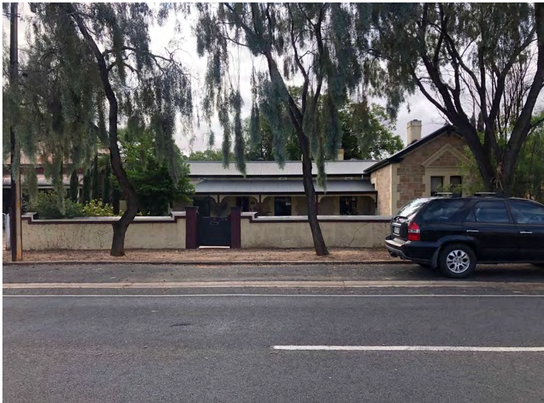
Dwelling and wall at 19 Second Street from south-east
