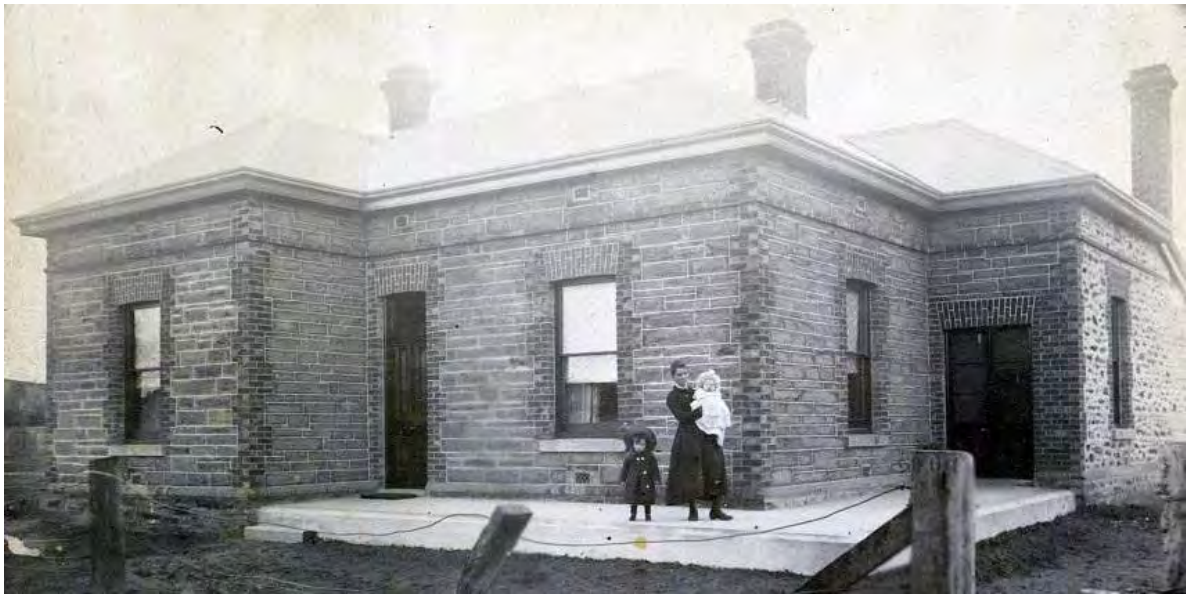
Home of James Forgie, 17 King Street, under construction, n.d. [Source: Taylor and Forgie]
