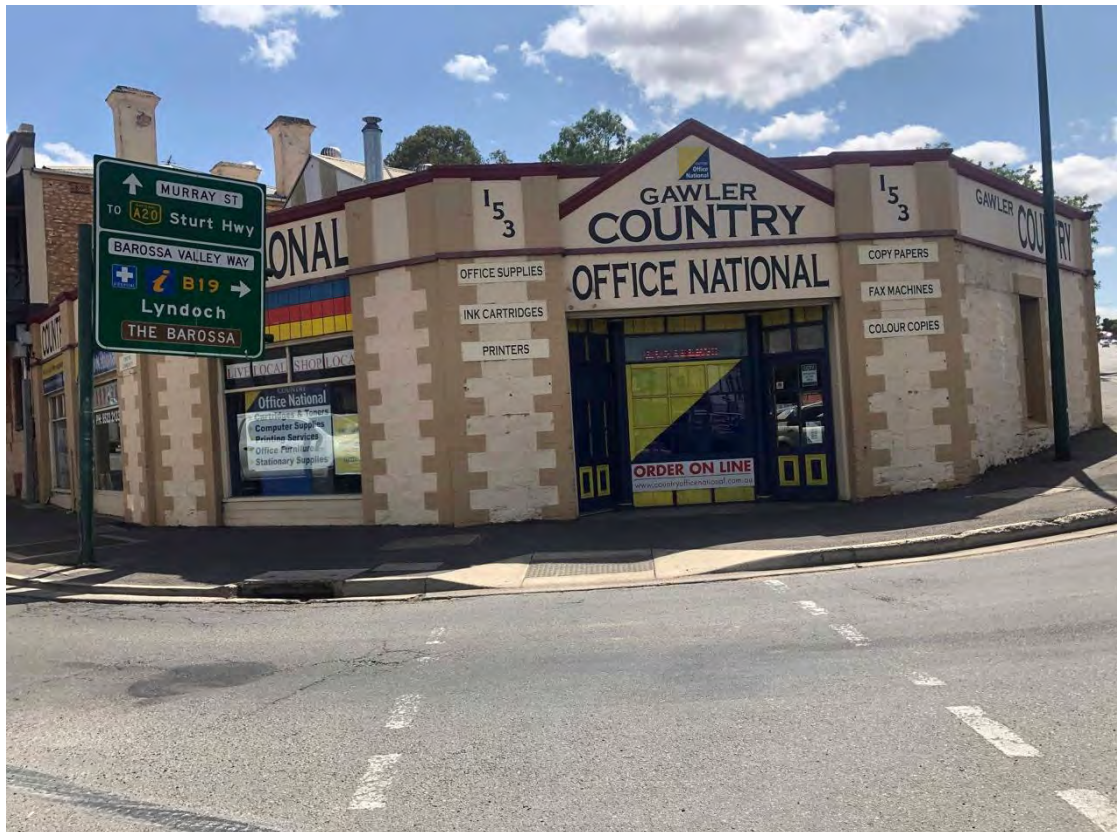
Corner workshop at 153 Murray Street from west
