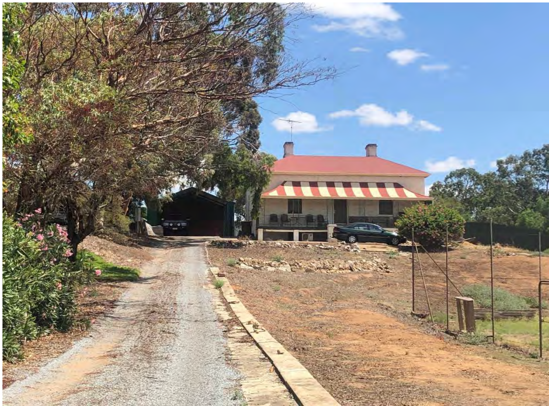
Dwelling at 30 Eighth Street from south-east
