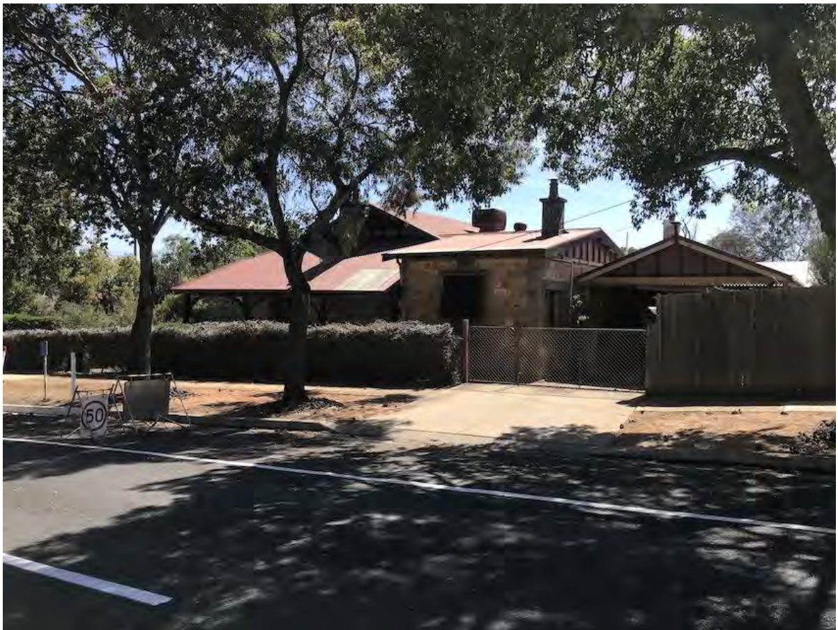
Dwelling at 47 Lyndoch Road from west
