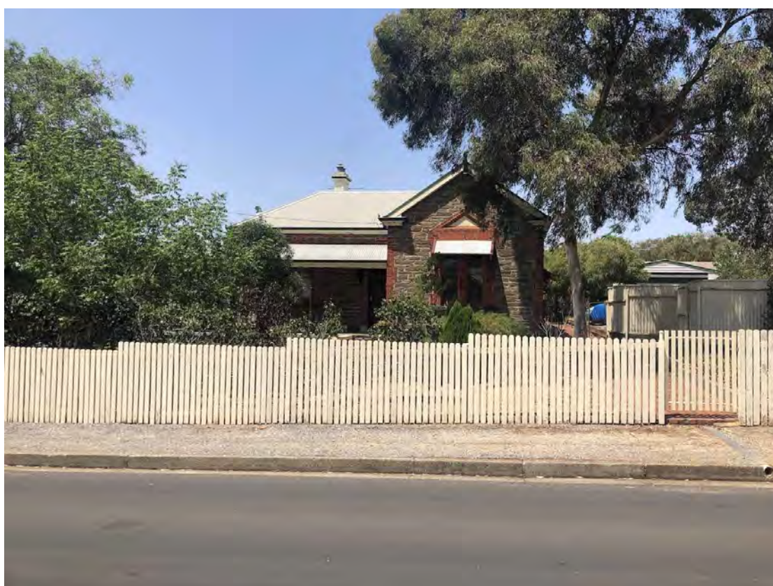
Dwelling at 13 Daly Street from west
