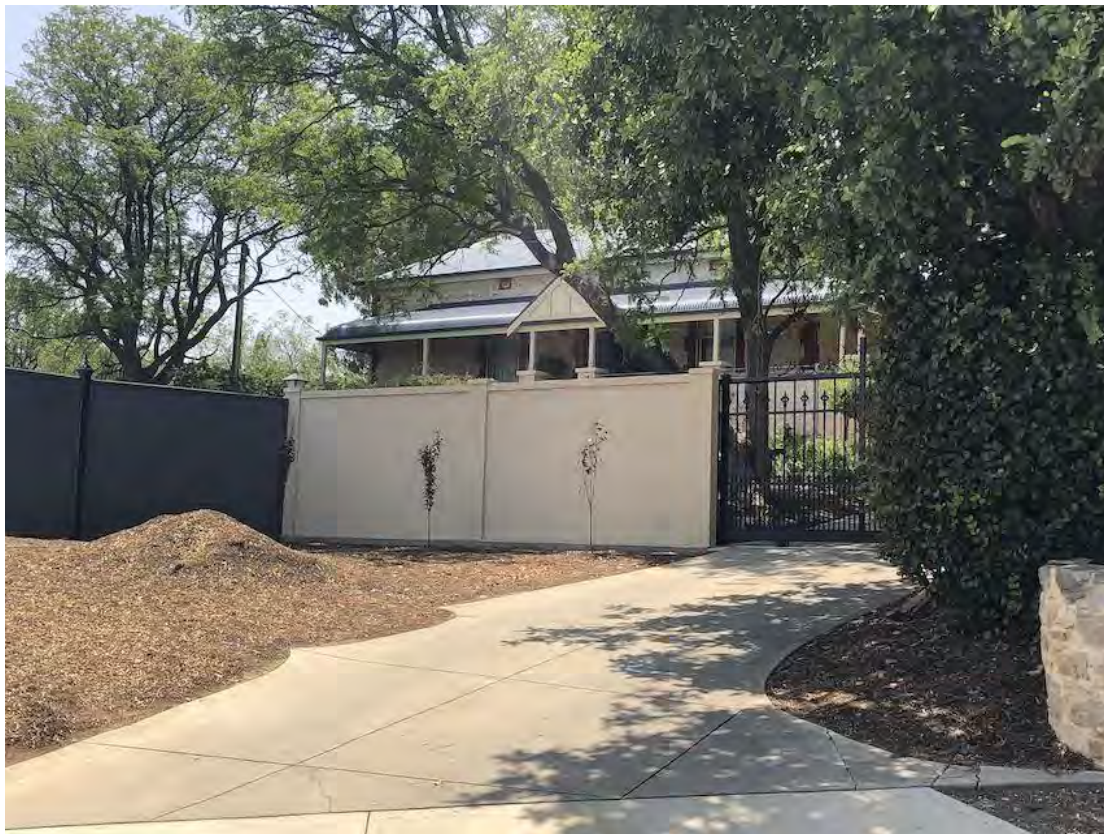
Dwelling at 11 Blanch Street from south-west
