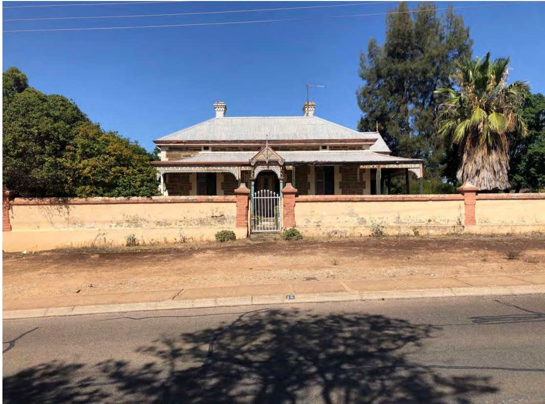
Dwelling and wall at 19 Thirteenth Street from west
