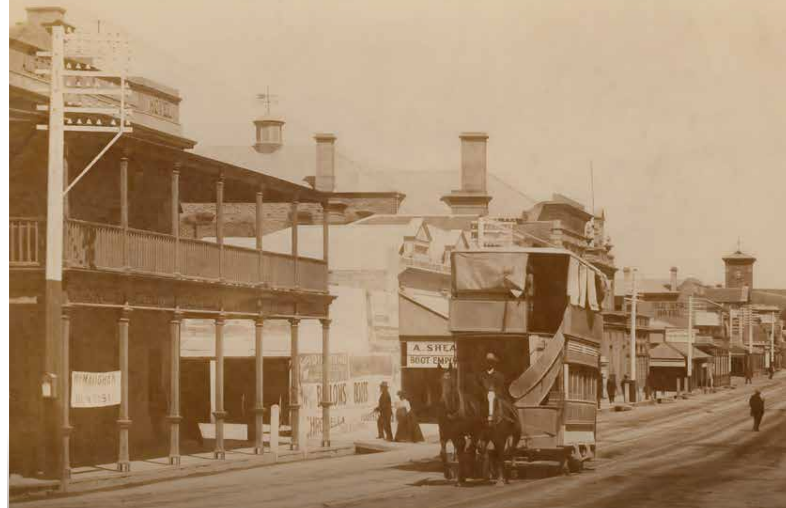
Figure 4. Historical Image Murray Street in Gawler Town Centre (Source: Phillips Pilkington)
