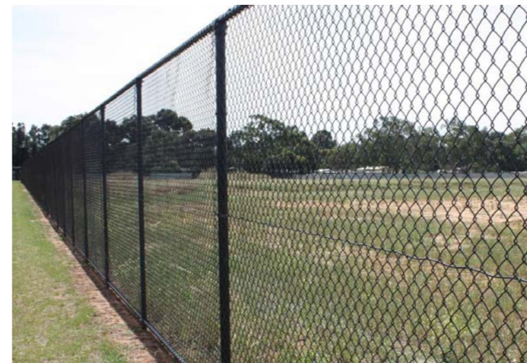
Chain Link Fence
