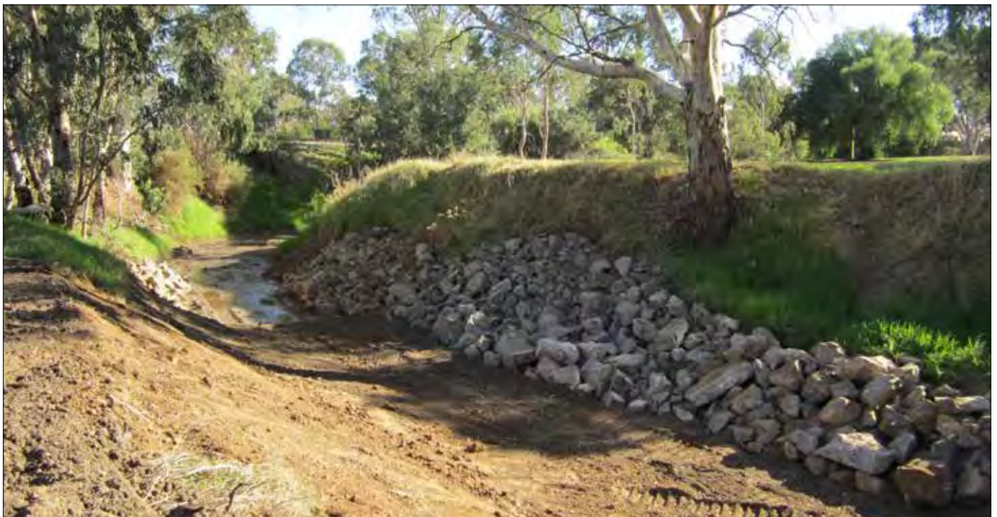
Placement of erosion rock for the Gawler Urban Rivers Biodiversity Program
