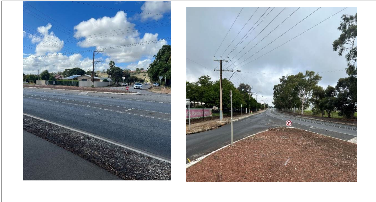
Figures 8A & 8B. Sherriff St junction with Main North Road
