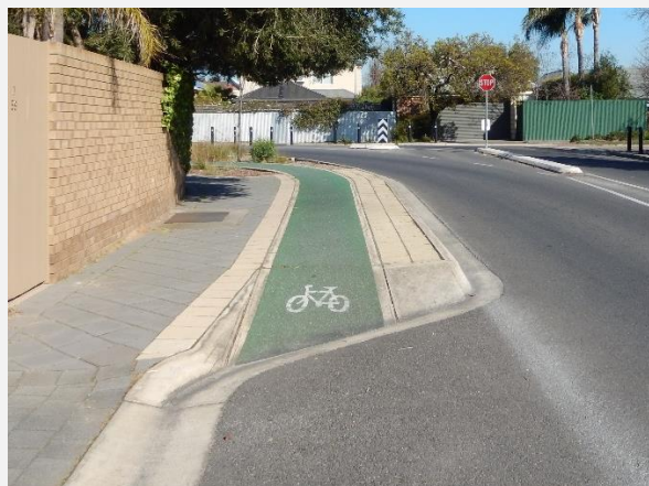
Figure 53: cyclist ramp up to footpath to avoid squeeze point
