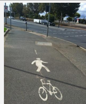
Photo 27: Section of footpath converted to shared path to access signalised crossing.
