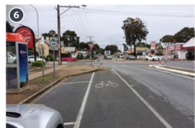
Photo 6: Potentially hazardous squeeze point for cyclists on Adelaide Road at Sixth Street intersection
