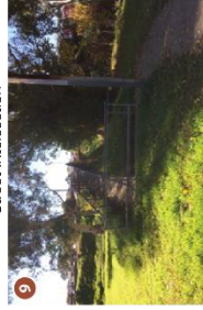
Photo 9: Approach angle and width of footbridge south of Whitelaw Terrace too steep/narrow for the high levels of cycling, pedestrian activity from shopping centre.
