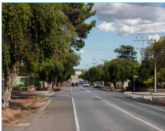
Main North Road Willaston – Road and Stormwater Upgrade
