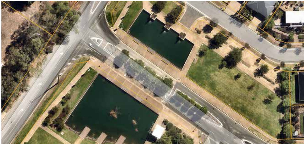
Figure 9. Ornamental lakes at Orleana Waters are part of a significant scale IWM project overseen by Council (source: Town of Gawler, 2025). Due to the challenges in staging of land releases between different owners as well as local geology, IWM concepts have been scaled back with each land release now to address stormwater impacts at the individual land division scale
